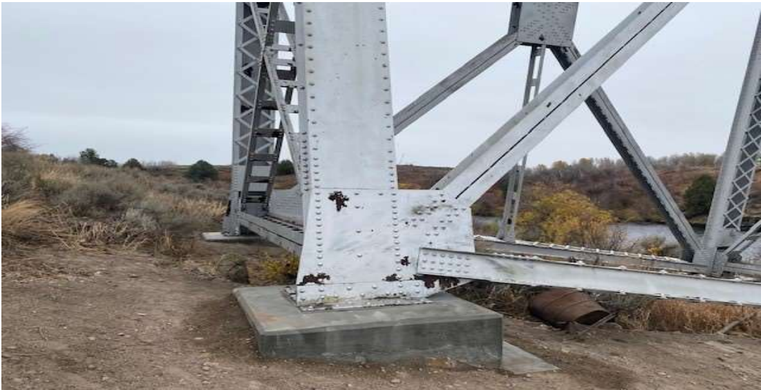
Fall River Bridge Footings
