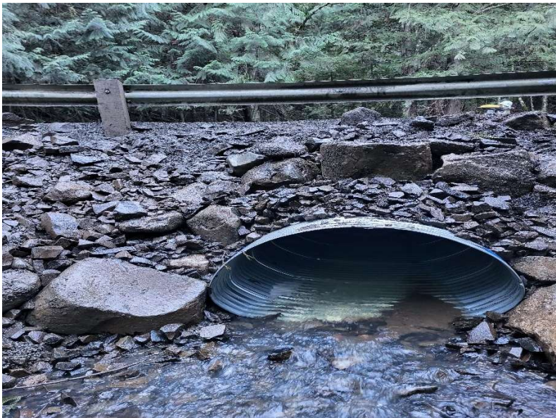
Dworshak Drift Creek Culvert
