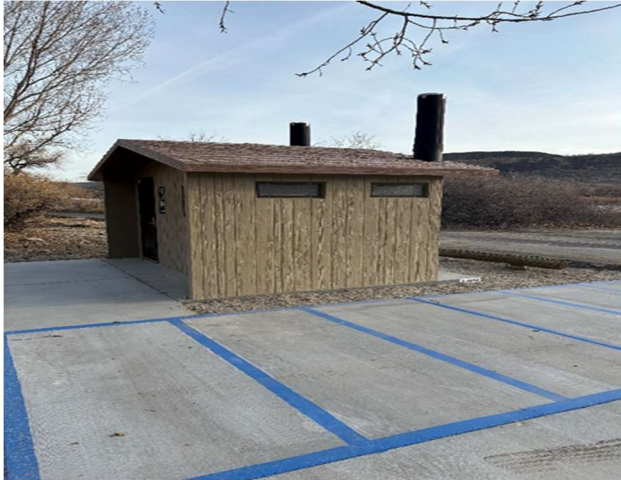
Box Canyon Vault Toilet
