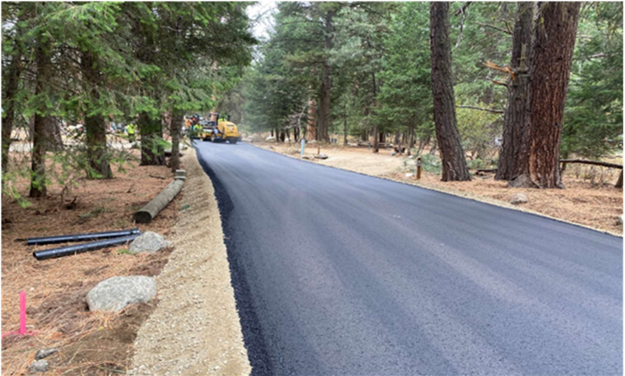
Chokecherry Loop Electric & Water Upgrades
