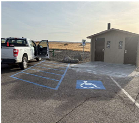
Box Canyon Vault Toilet
