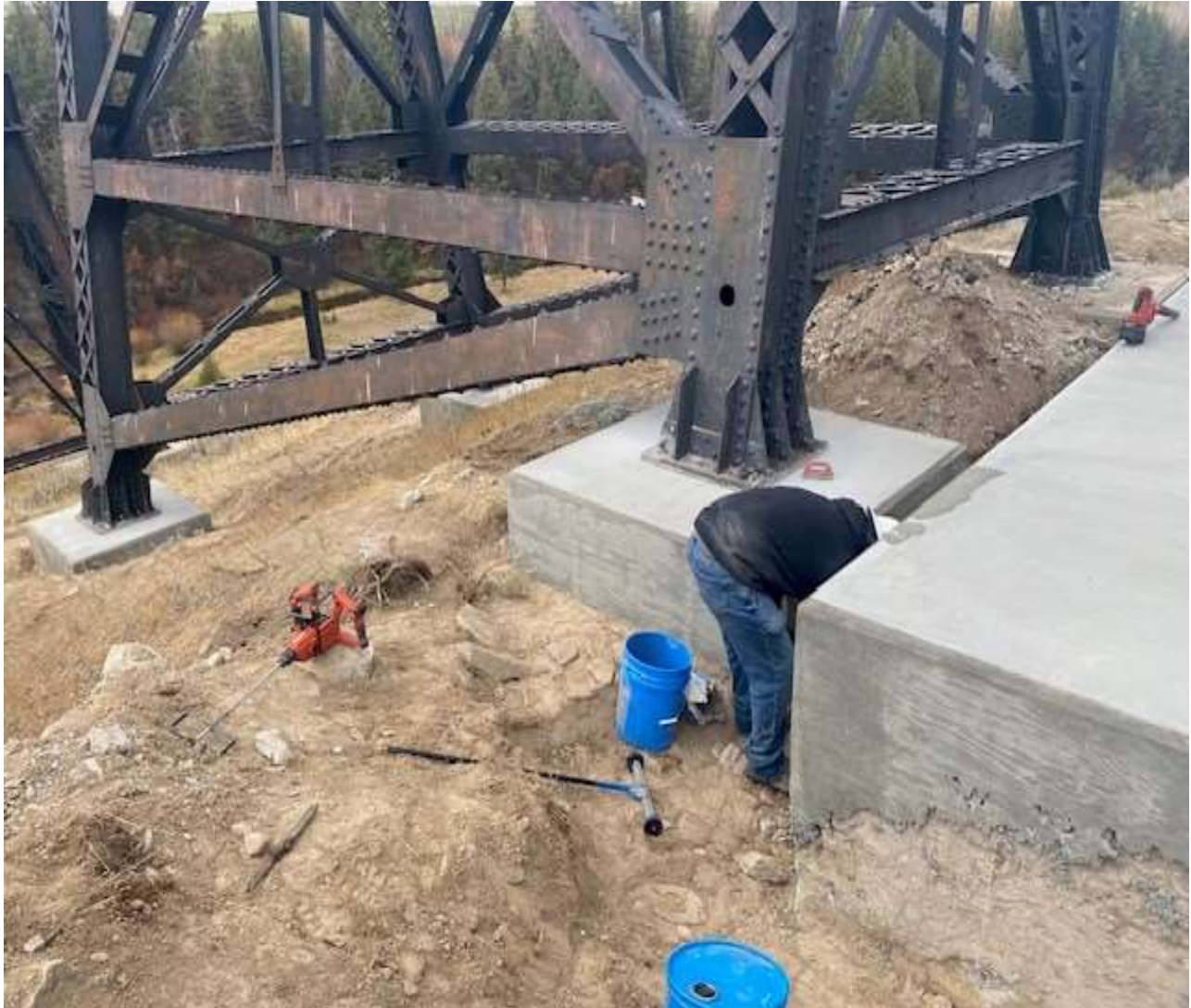
Conant Bridge Footings
