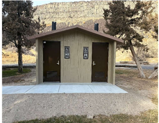
Niagara Springs Vault Toilet
