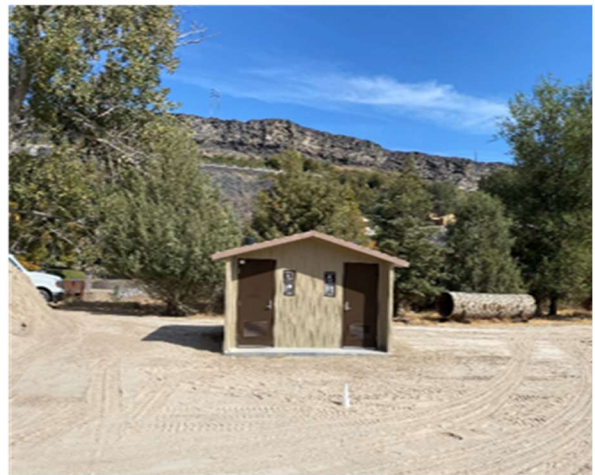
Ritter Island Vault Toilet
