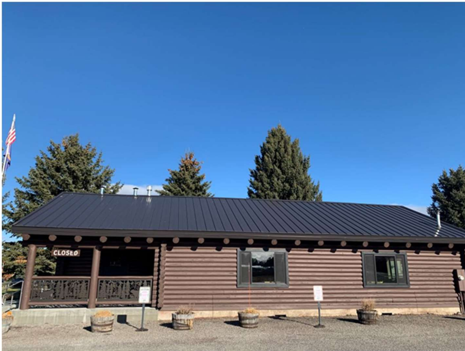
Ashton Tetonia Visitor Center New Roof
