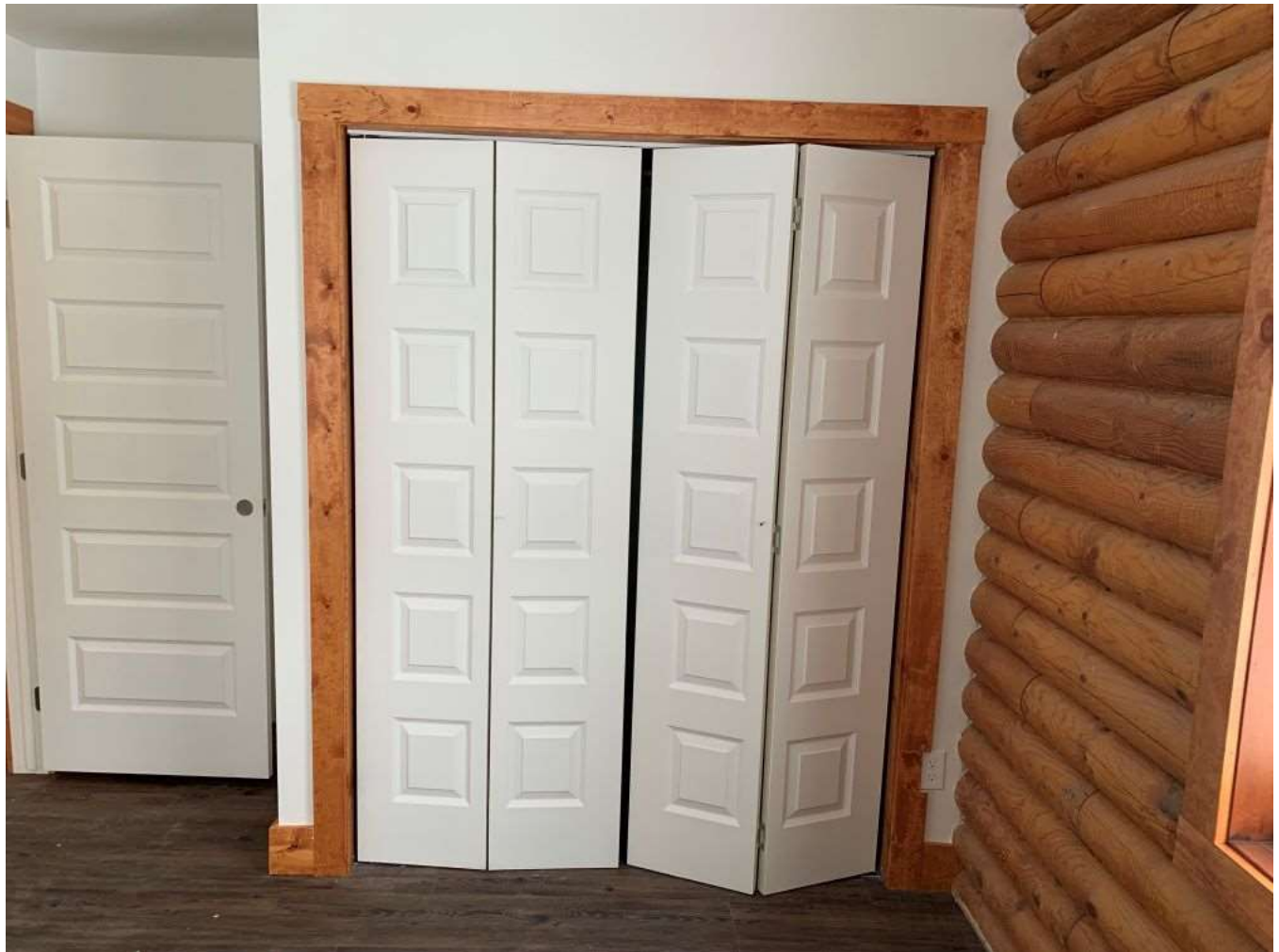
Henrys Lake Staff Cabin Repairs
