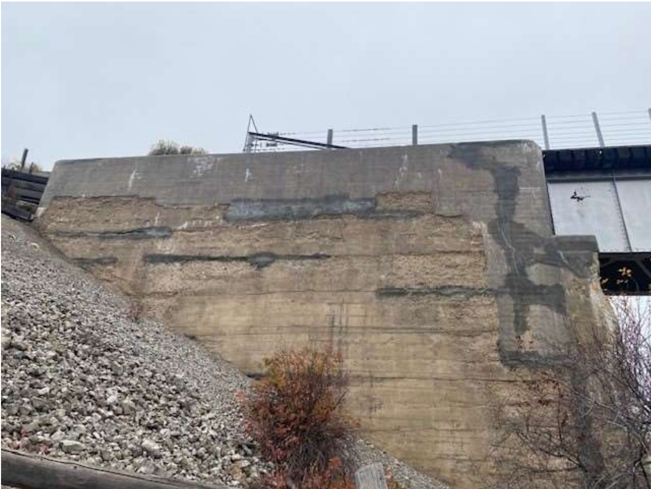
Fall River Bridge Repairs
