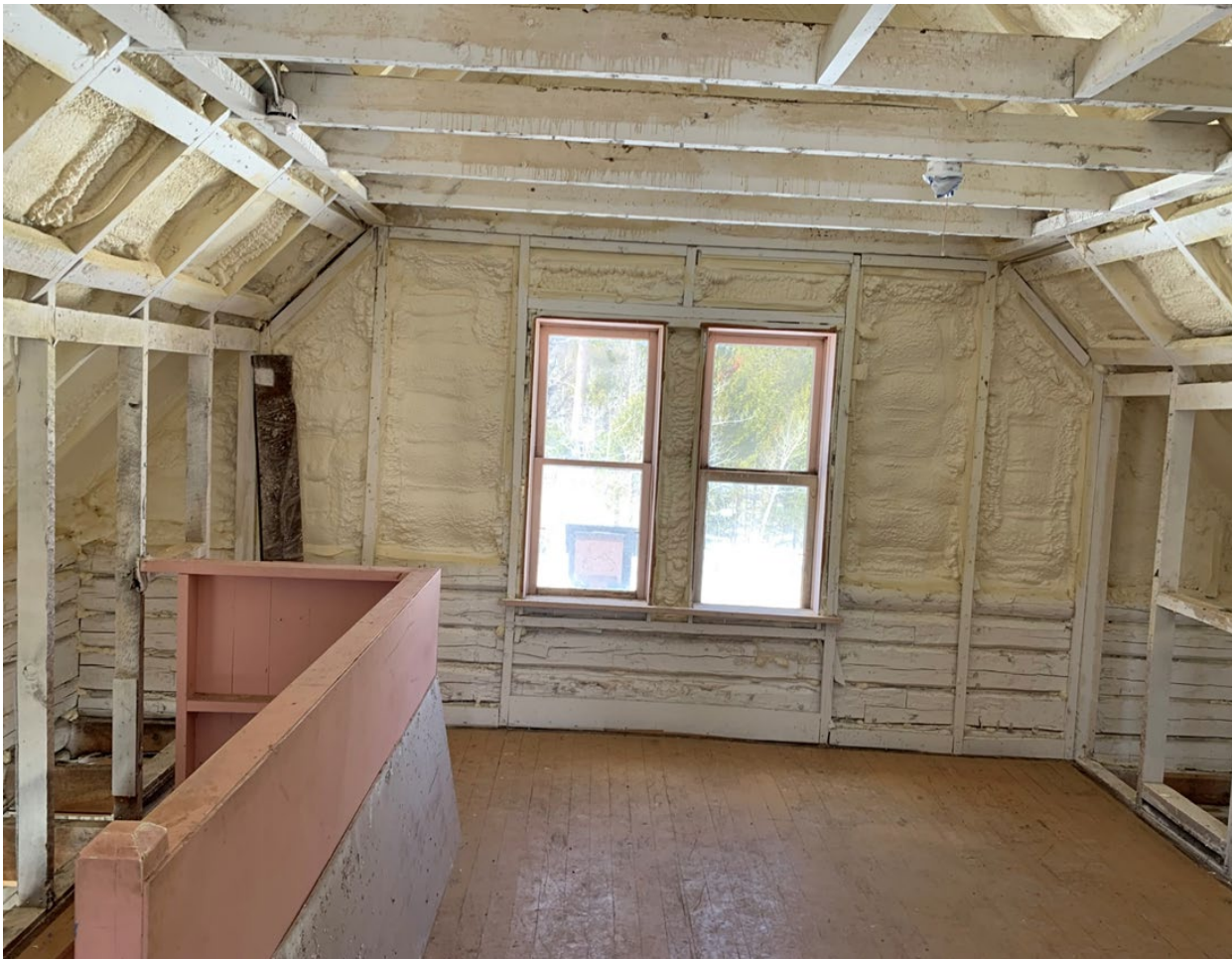
Harriman Honeymoon Spray Foam Installation
