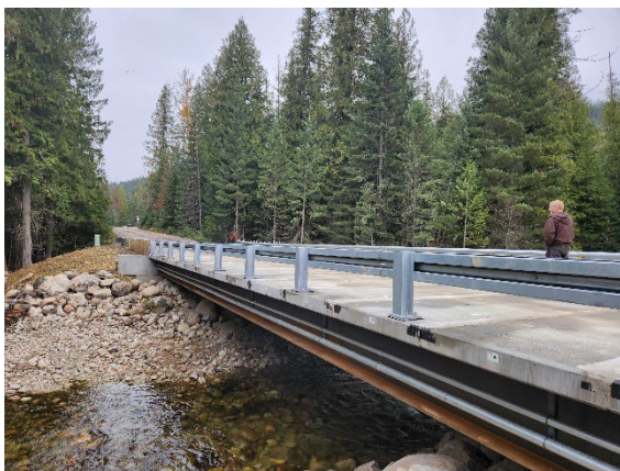
New Bridge built by IDL near Lionhead Unit of Priest Lake State Park. Park Manager Lonnie Johnson showing his excitement.
