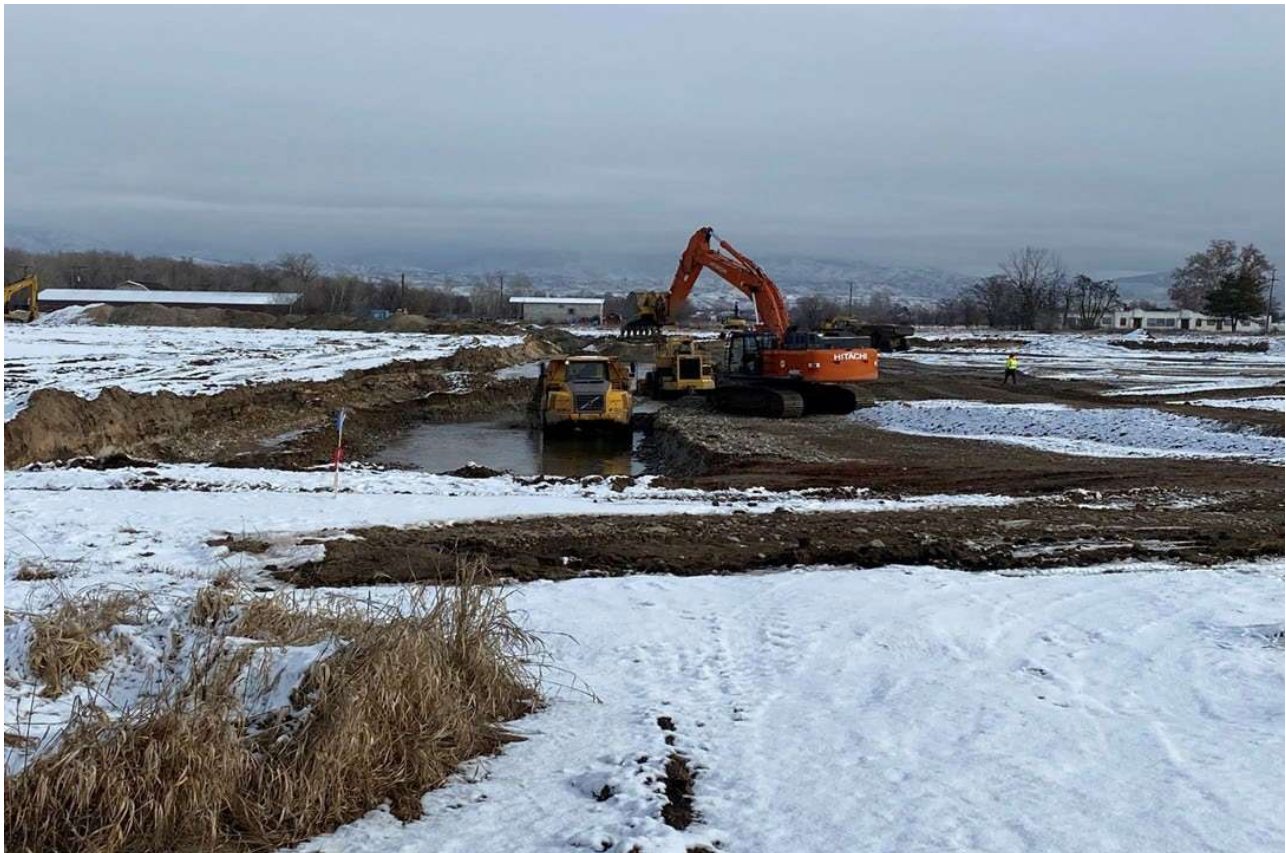
Eagle Island RV Campground – Excavating Pond
