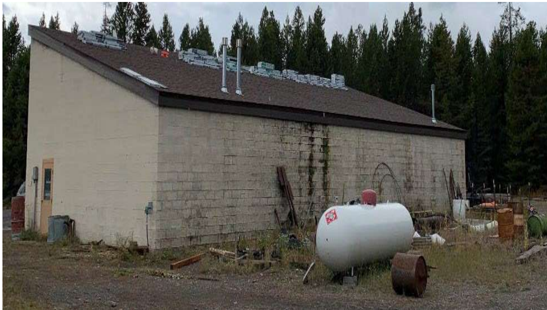
Harriman Gas Storage Maintenance - Surplus
