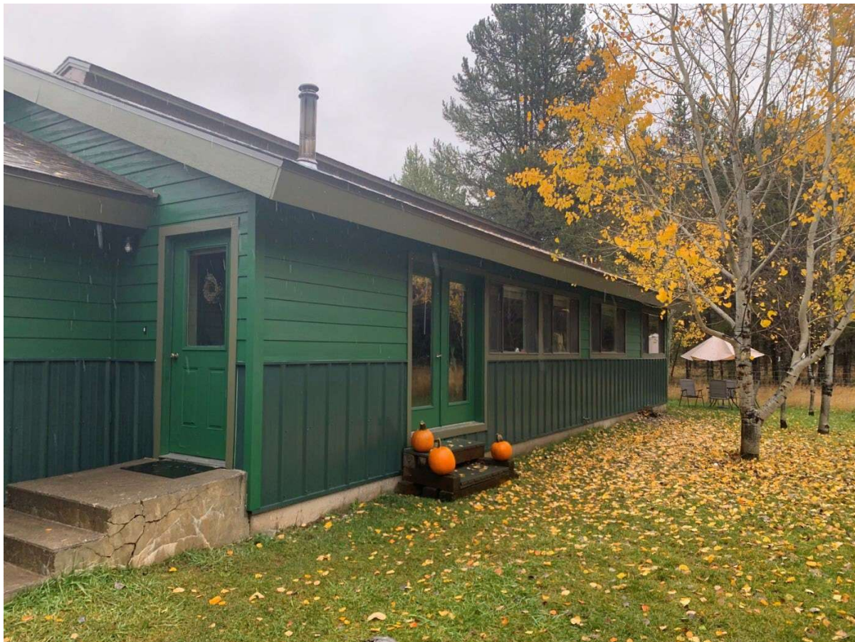
Harriman Manager’s House Maintenance
