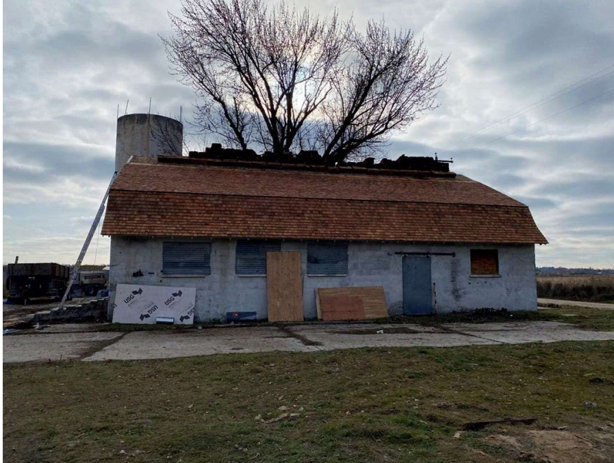
Eagle Island Dairy Barn Reroofing
