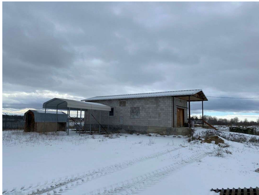
Eagle Island Storage Building Reroofing
