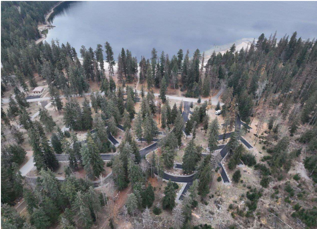
Priest Lake Campground Electrical Upgrades
