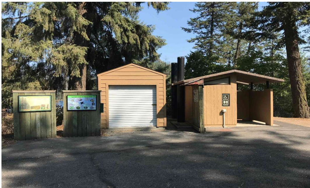
CDA Parkway Rehabilitate & Vault Toilets
