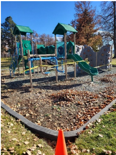
Finished Playground Curbing
