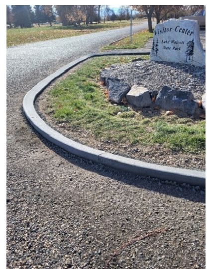
Finished Parking Lot Curbing
