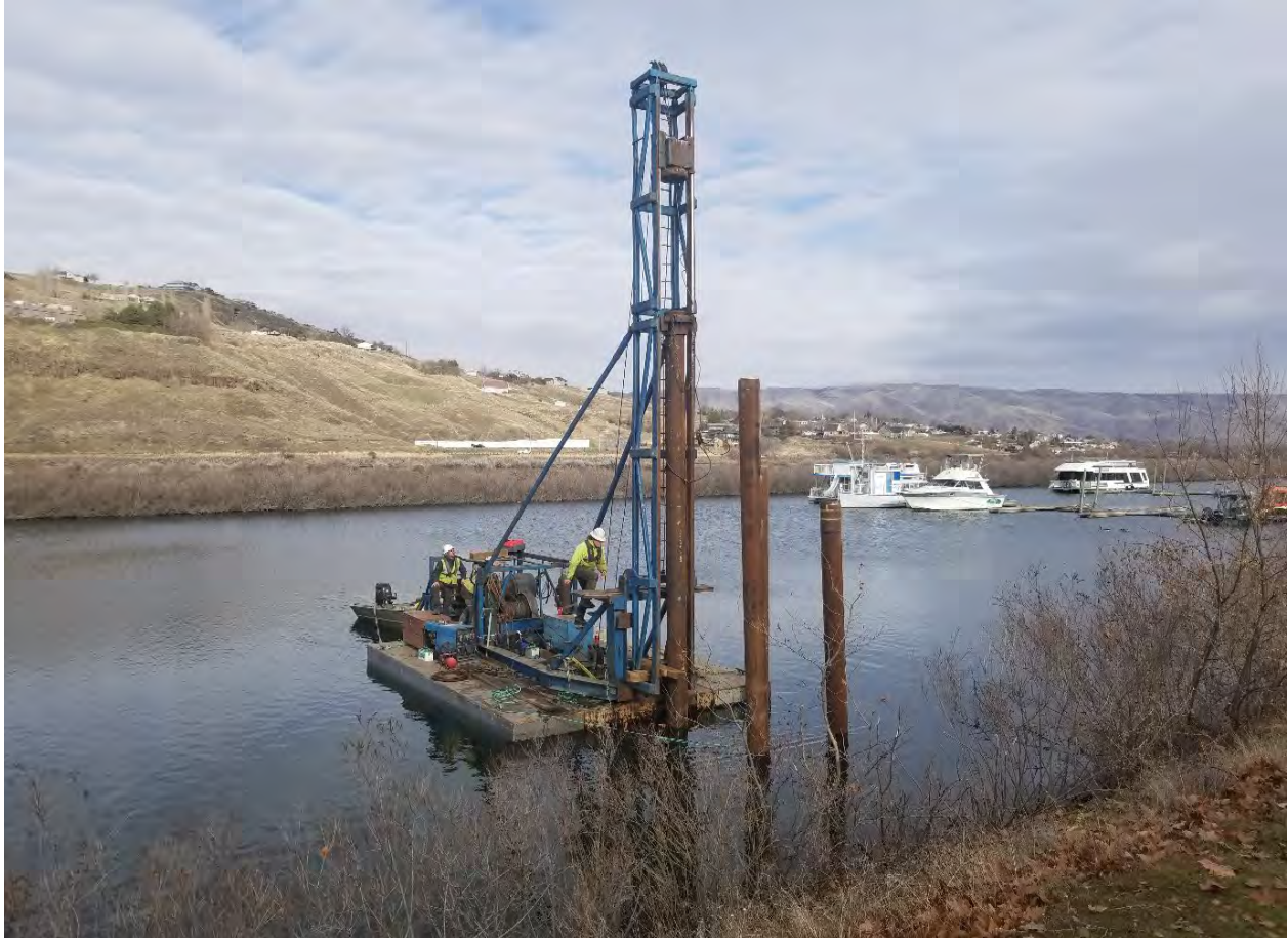
Hells Gate Marina Mooring Dock Replacement
