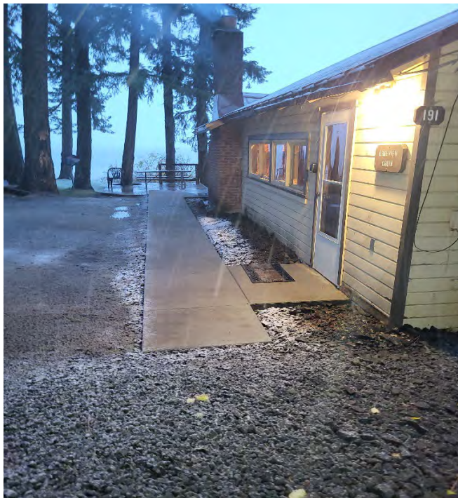
Heyburn Lake View Cottage New Walkway
