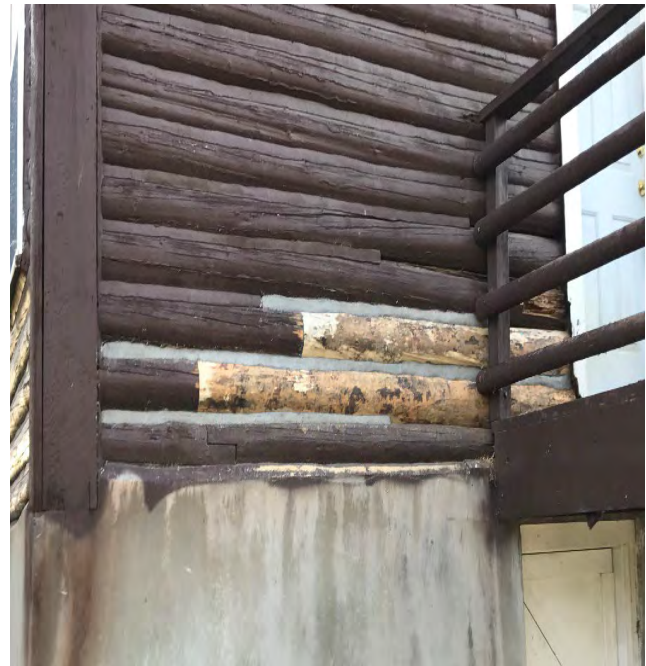
Ranch Office Log Repairs - After
