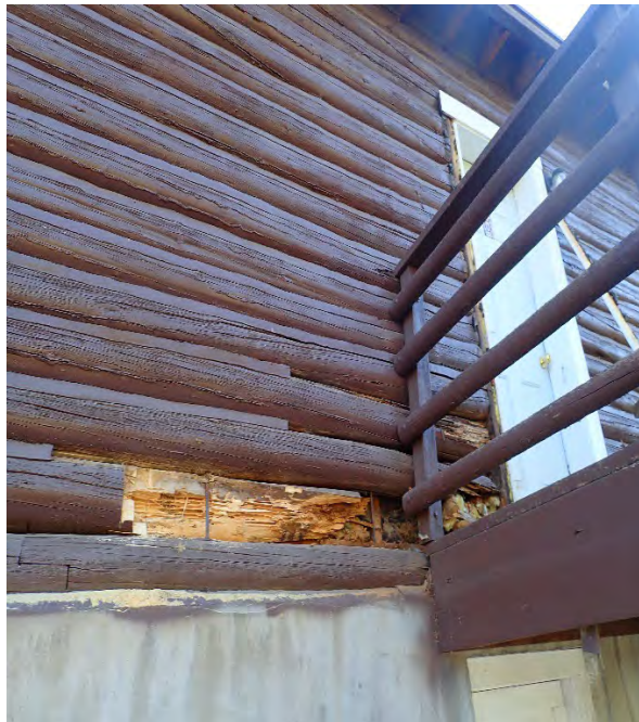
Ranch Office Log Repairs – Before
