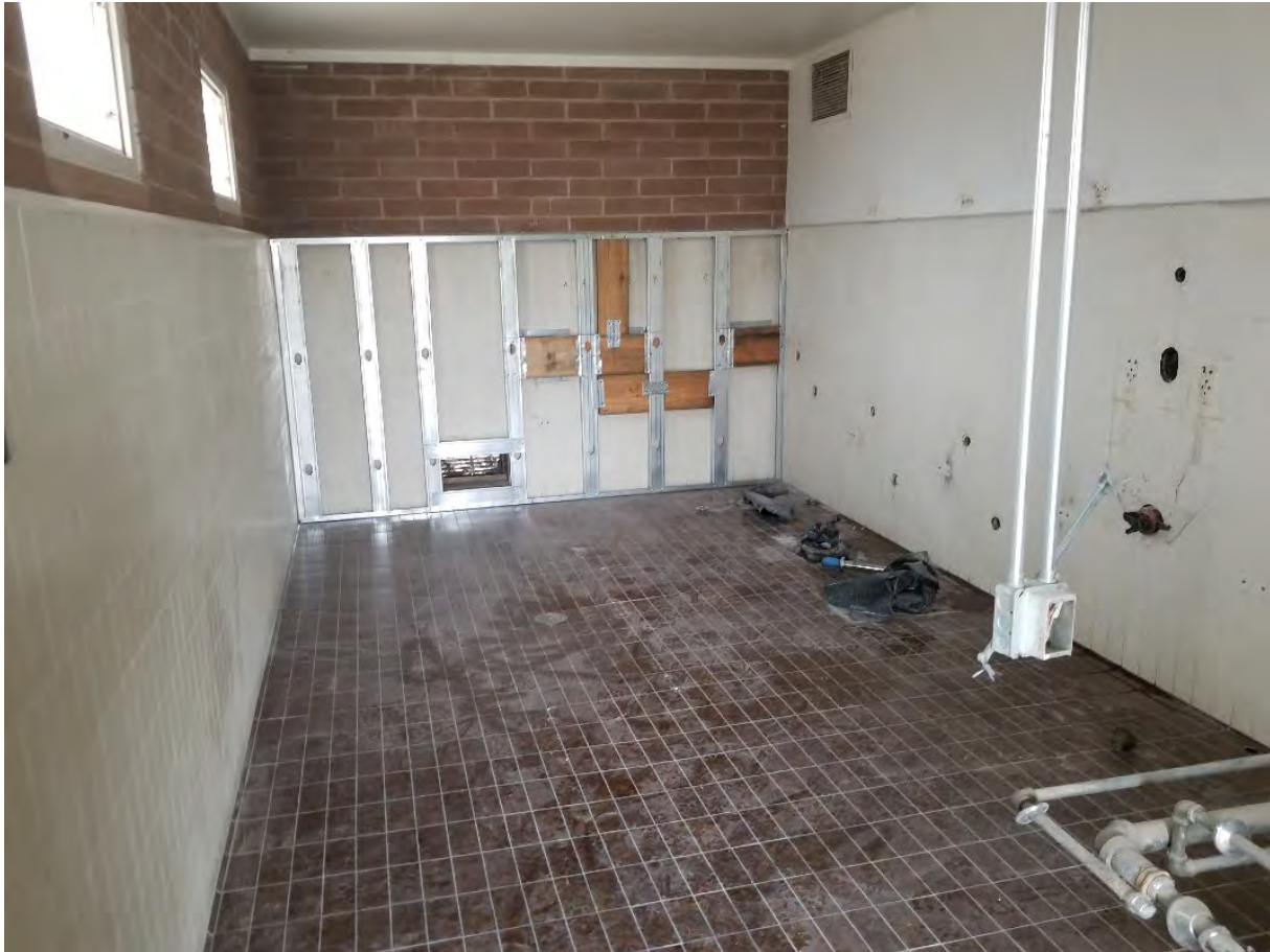
Hells Gate Remodel Marina Restroom
