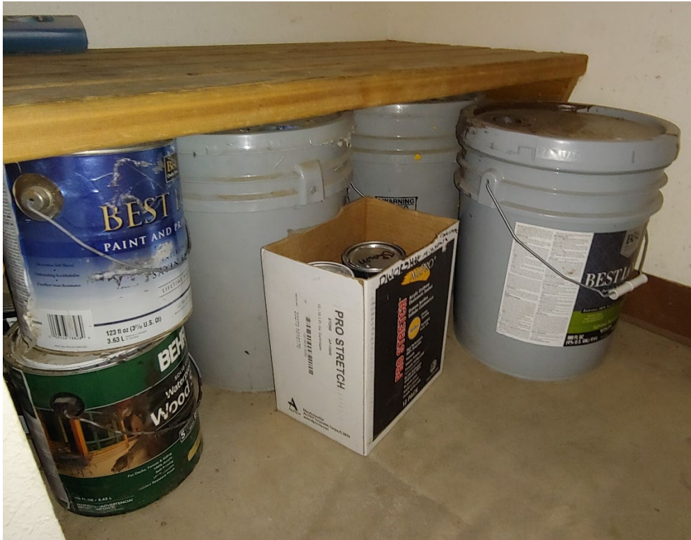
Figure 15-17. Paint stored on the floor of the bathroom in the Freeman Creek Campground maintenance garage
