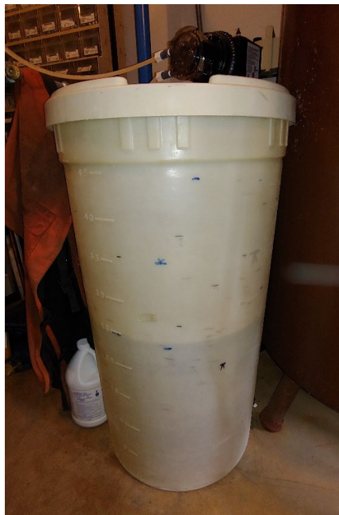
Figure 15-39. Unlabeled 45-gallon chlorine tank inside the Three Meadows Group Camp surface water treatment facility
