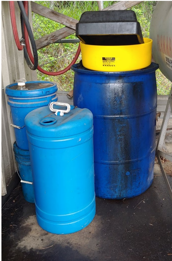
Figure 15-14. Used oil disposal drum with oil drips at the Freeman Creek Campground maintenance area
