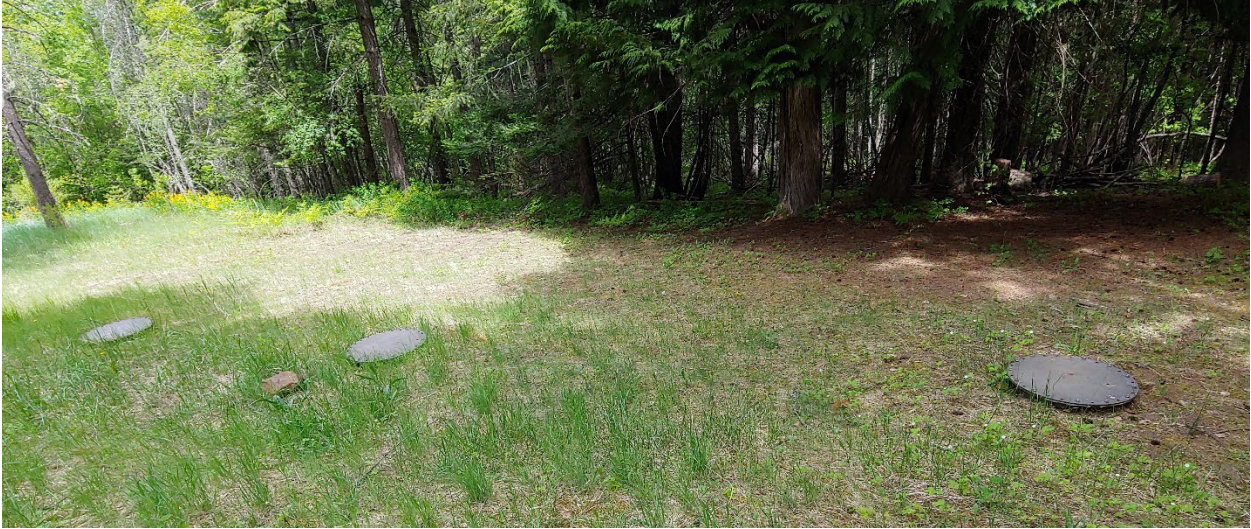
Figure 15-42. Three Meadows Group Camp 3,000-gallon septic tank
