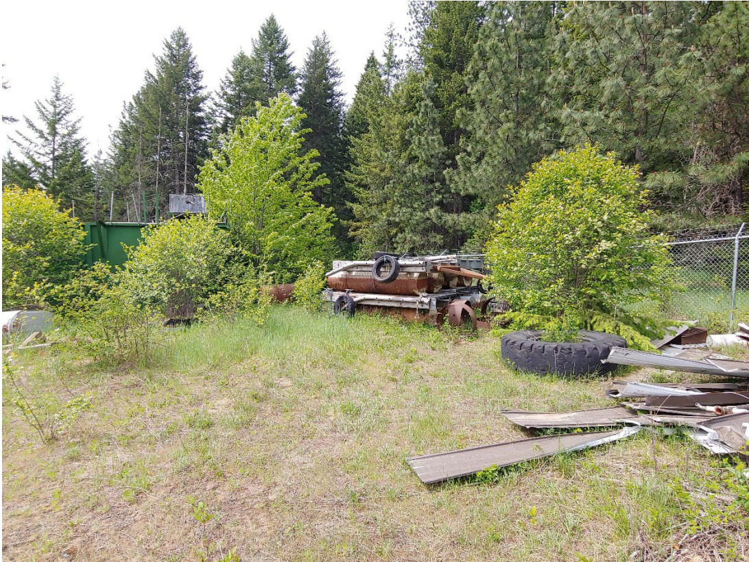
Figure 15-32. Rubber tire and other scraps inside the sewage lagoons enclosure at Freeman Creek Campground
