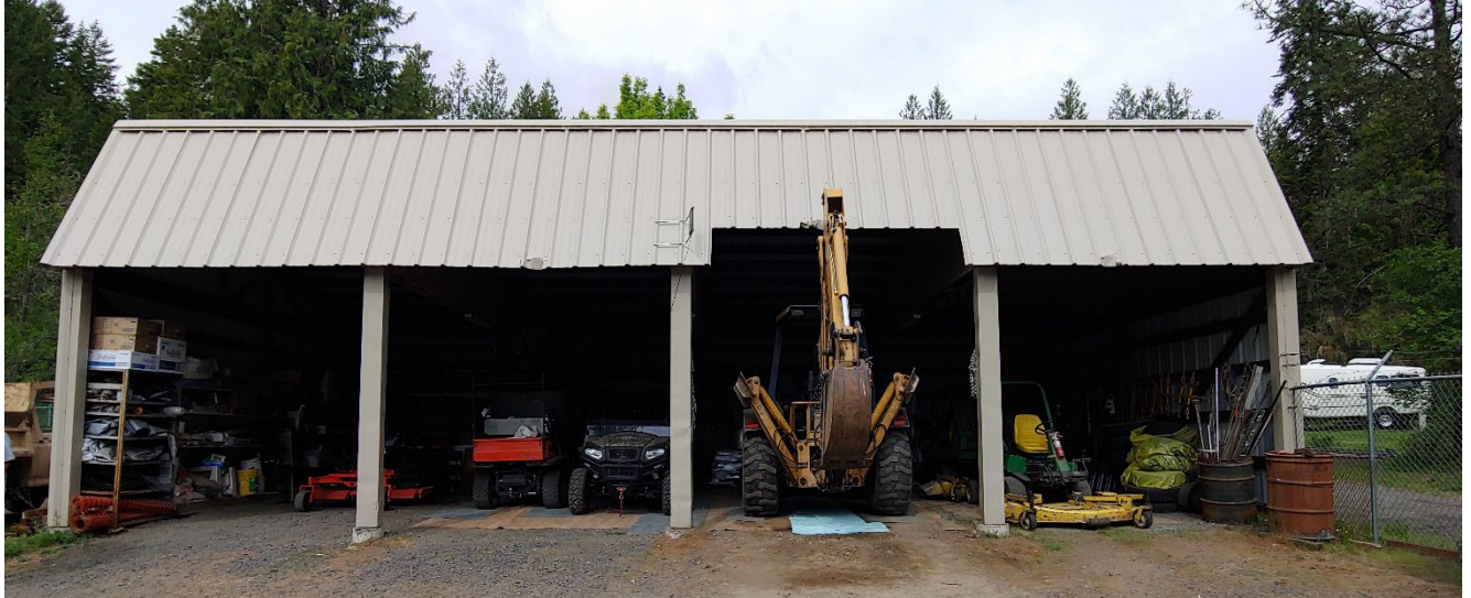
Figure 3-9. Freeman Creek Campground Vehicle Storage Shed
