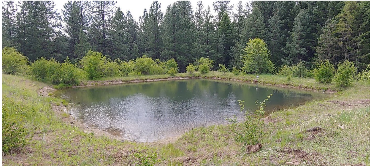
Figure 15-30. Smaller sewage lagoon at Freeman Creek Campground
