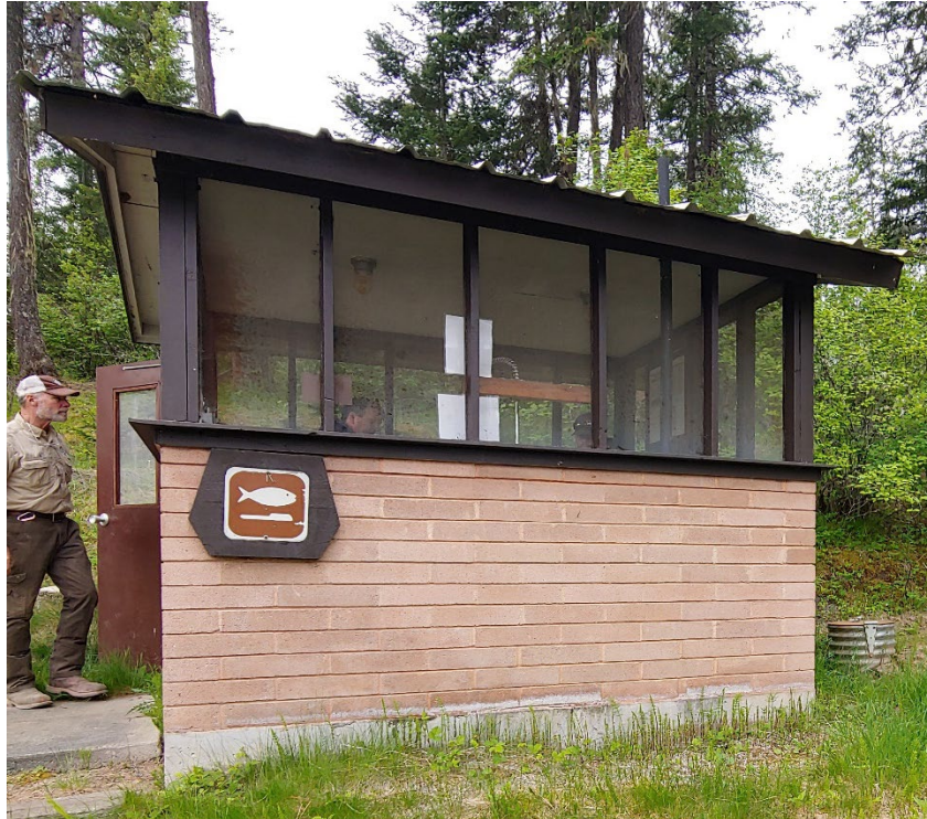
Figure 3-5. Freeman Creek Campground Fish Cleaning Station
