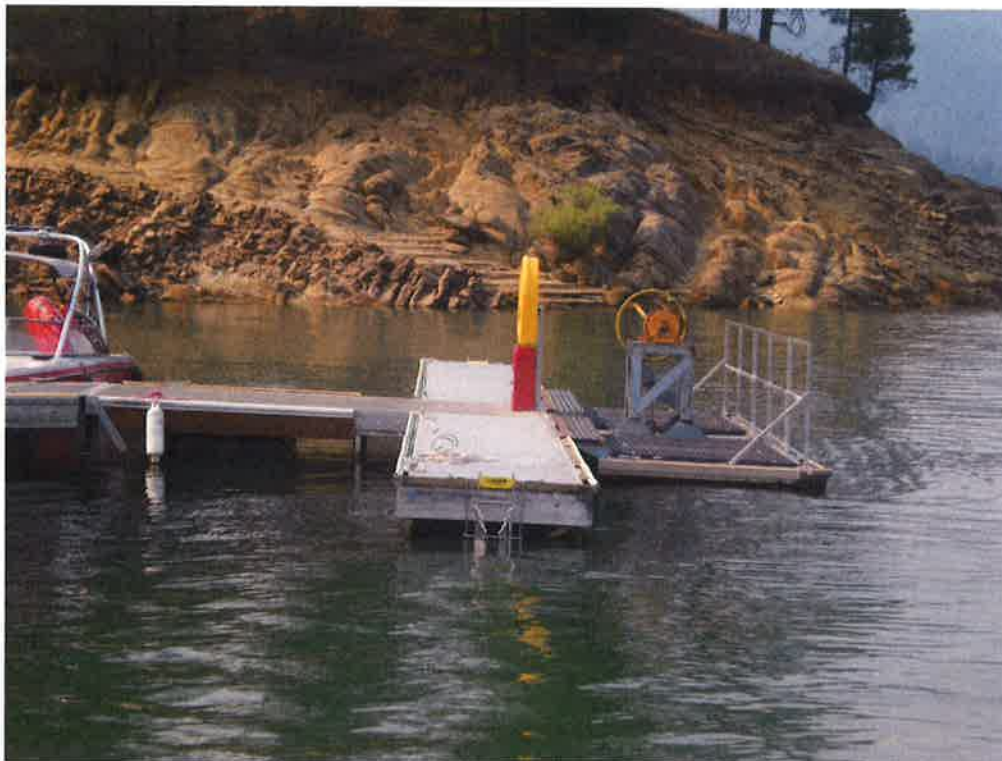
Figure 8 – Winch platform flotation deficiency
