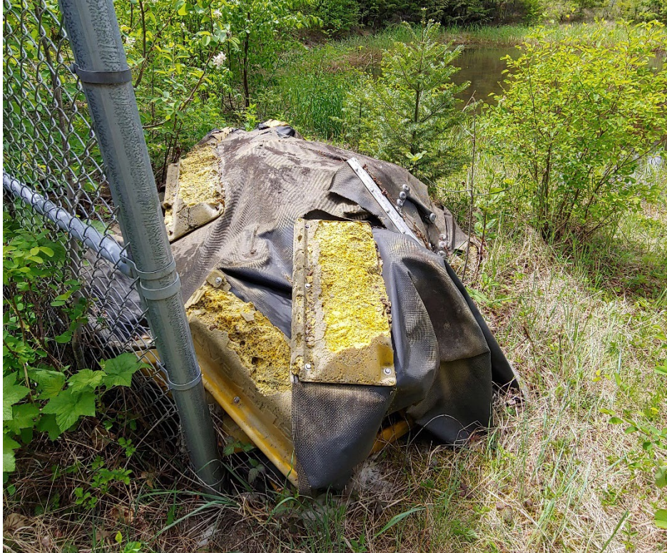
Figure 15-46. Discard cushion material inside the Three Meadows Group Camp sewage lagoons enclosure
