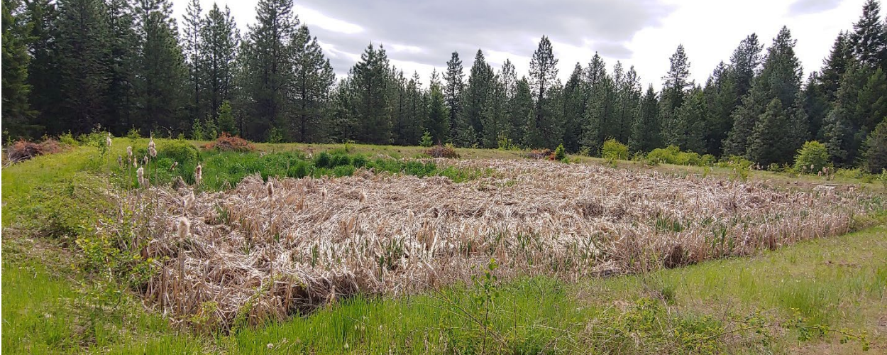
Figure 15-29. Larger sewage lagoon at Freeman Creek Campground with wetland vegetation
