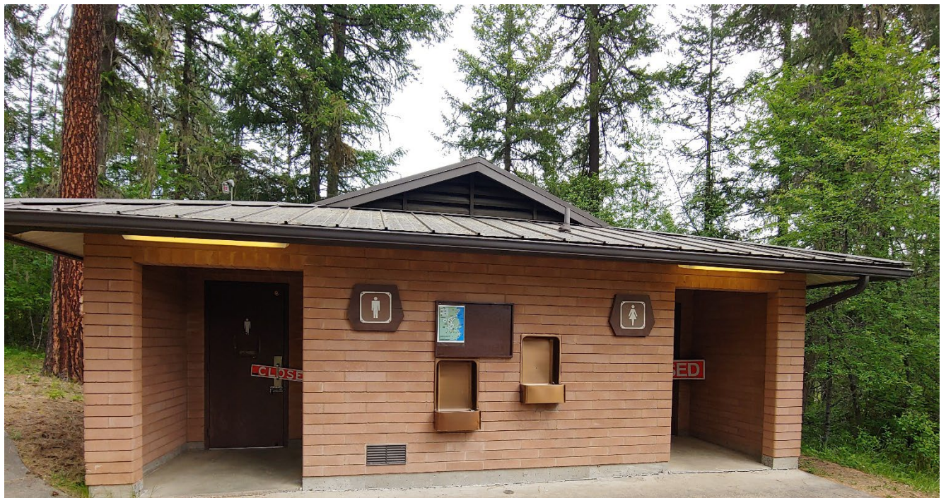
Figure 3-6. Freeman Creek Campground Plumbed Day Use Area Bathroom
