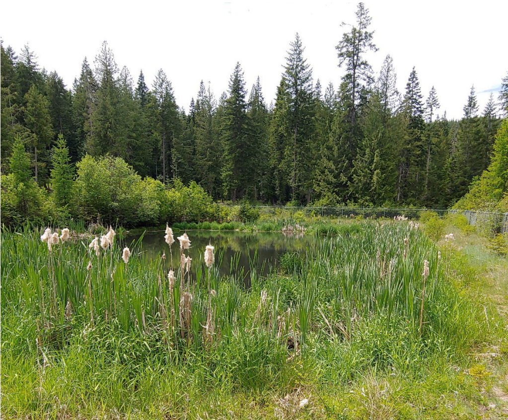
Figure 15-43. Three Meadows Group Camp sewage lagoon with wetland vegetation around the perimeter
