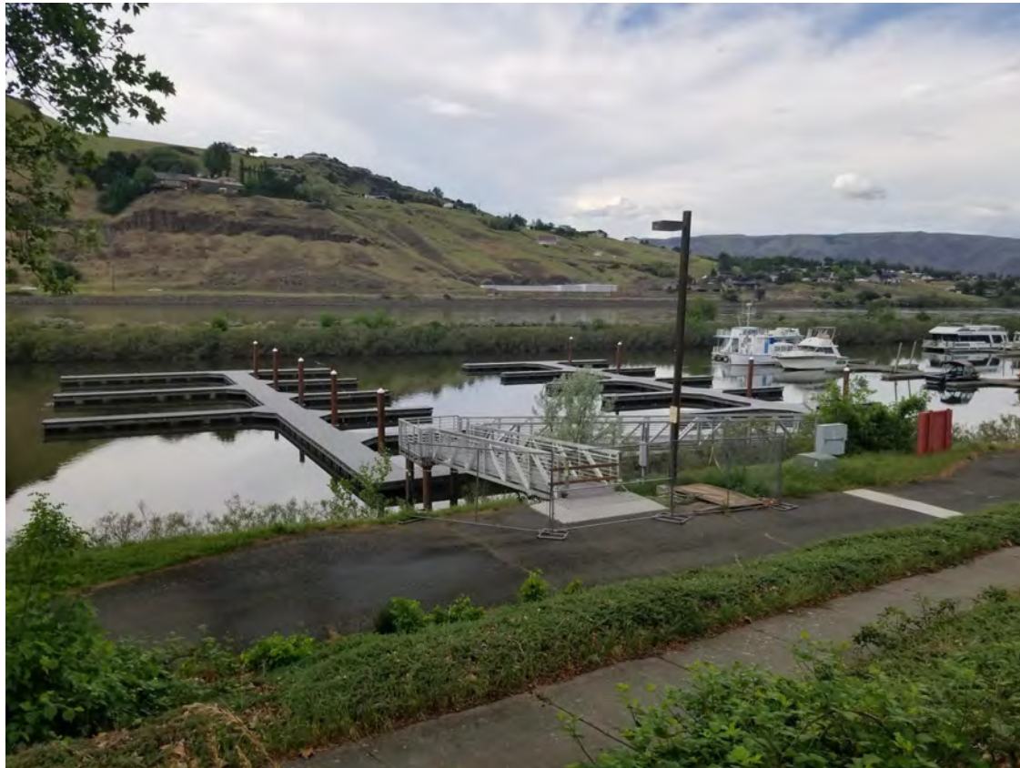
Hells Gate Marina Mooring Dock Replacement
