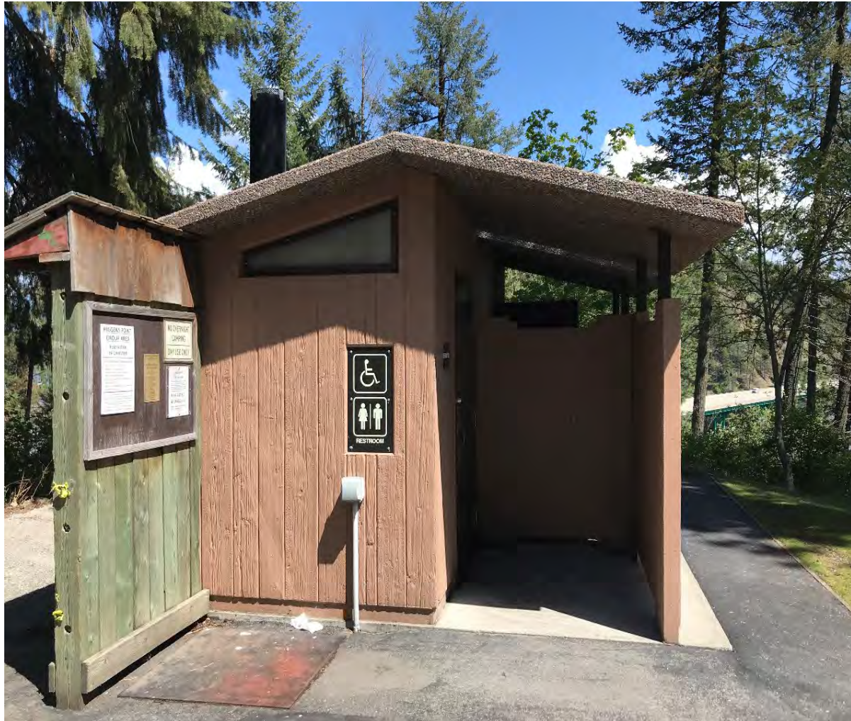
CDA Parkway Rehabilitate Vault Toilet
