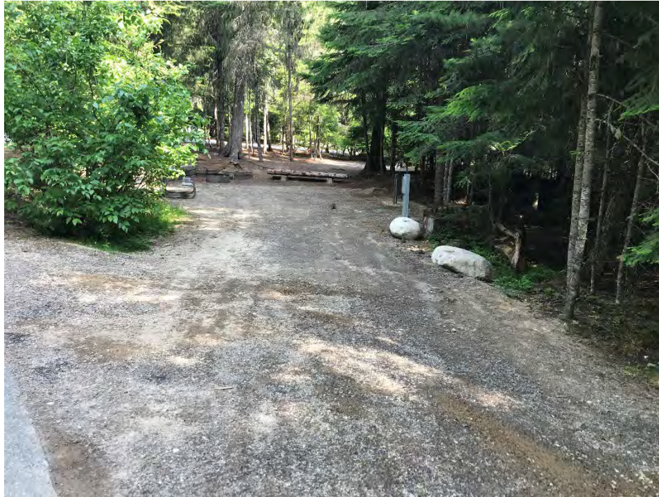
Priest Lake White Pine Electrical Upgrades
