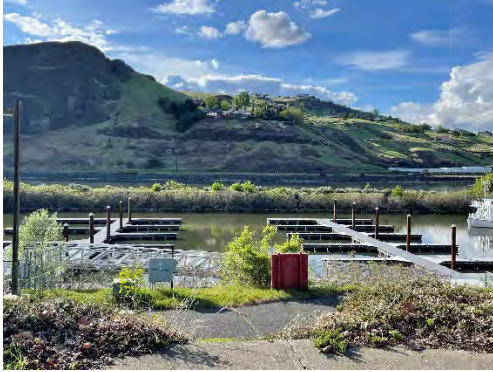
Hells Gate Dock upgrades looking good
