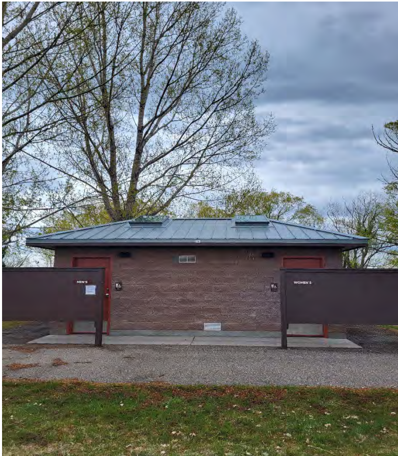
Lake Walcott Boat Ramp RR Repairs
