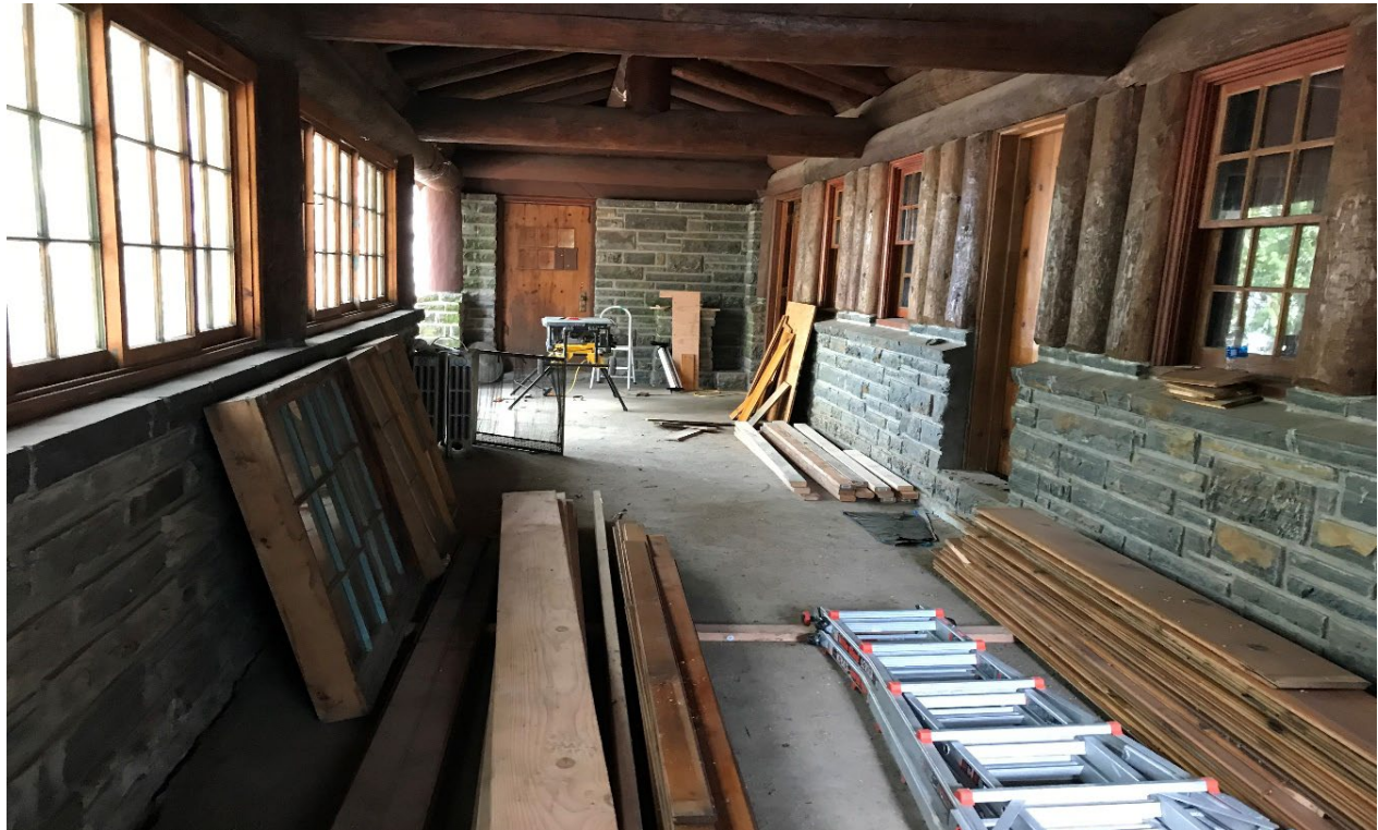
Heyburn Lodge Remodel
