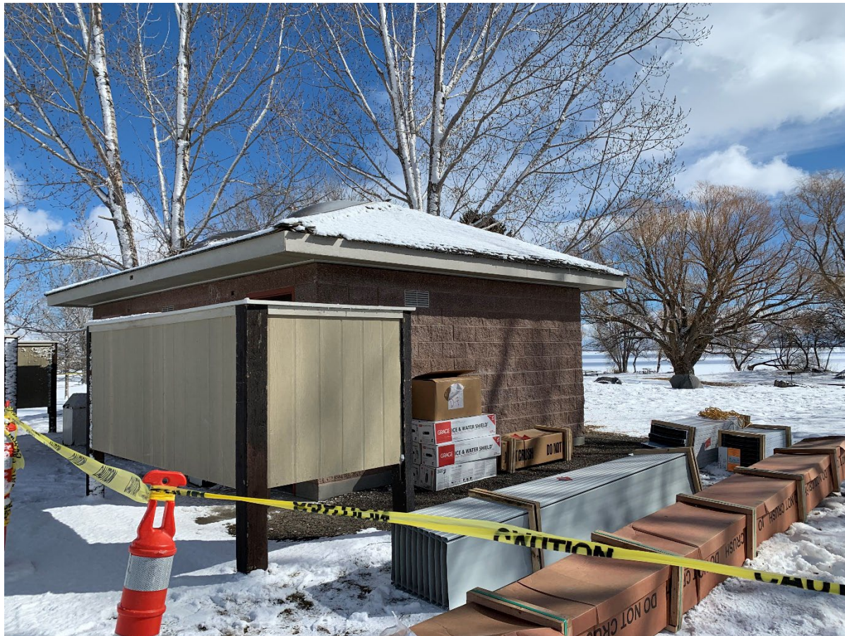
Lake Walcott Boat Ramp Restroom
