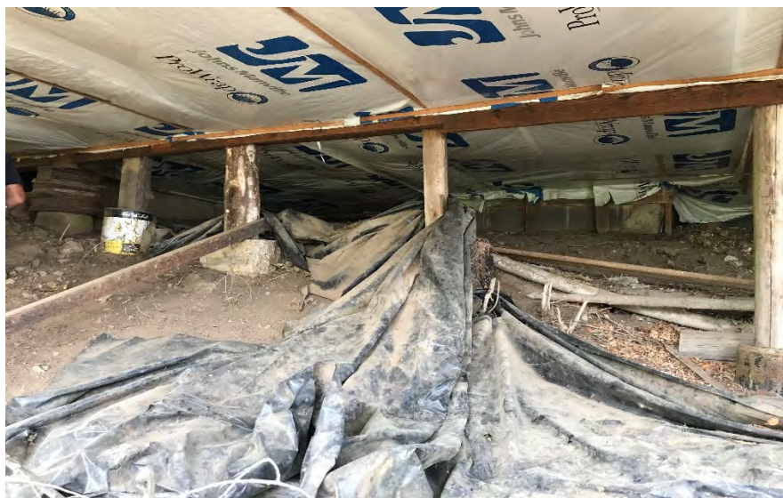
Heyburn Replace Lake View Cottage Foundation – Existing Foundation
