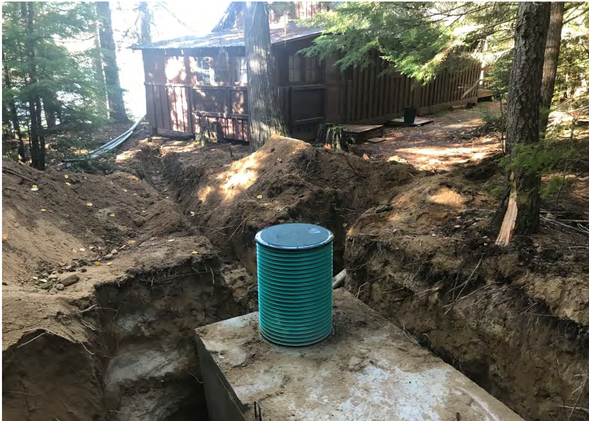
Priest Lake Shafer Cabin Elec & Plumbing Repairs – New Septic Tank
