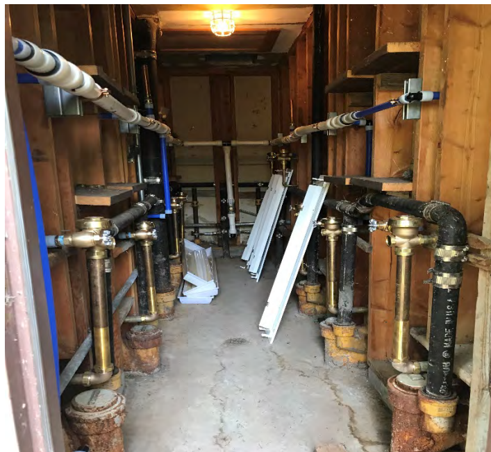
Dworshak Upgrade Shower House Plumbing
