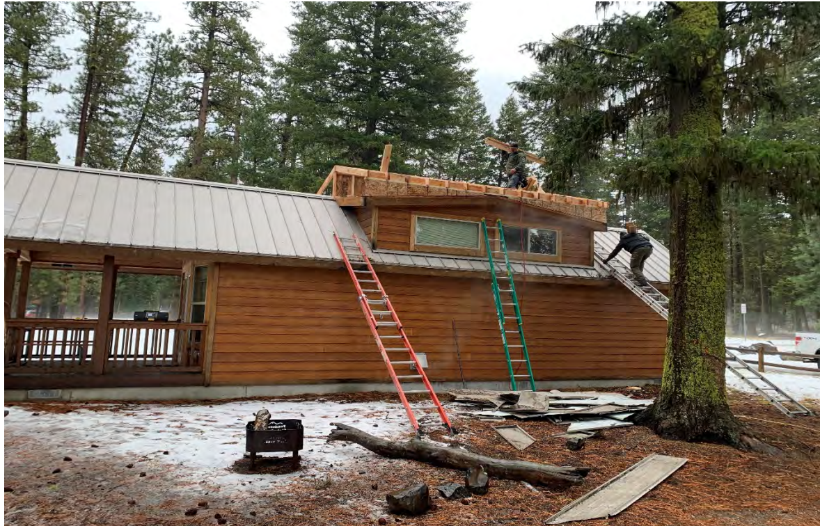
Ponderosa Re-Engineer Lakeview Cabin Roof Structures – Roof Reframing Under Construction
