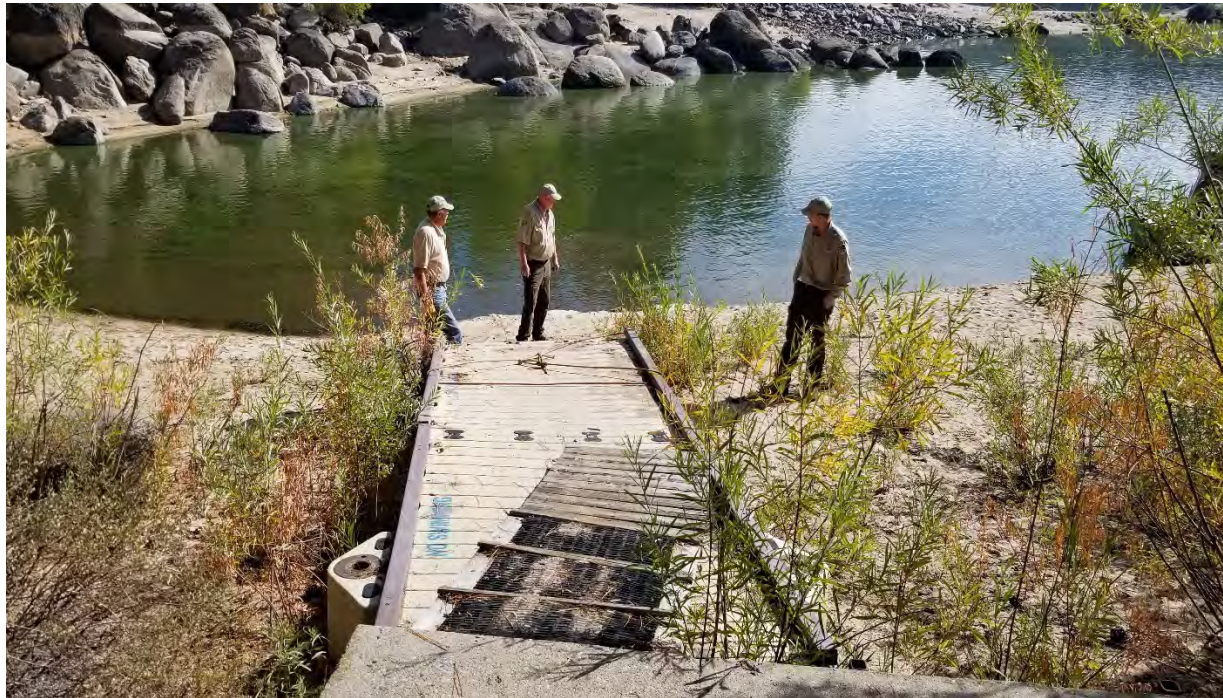
Lake Cascade Crown Point Docks – Existing Condition
