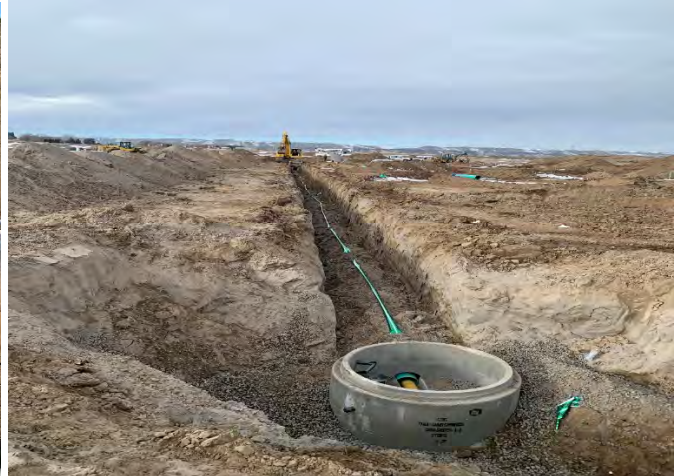
Thousand Springs Billingsley Creek Campground - On-site Materials & Sewer Line Installation
