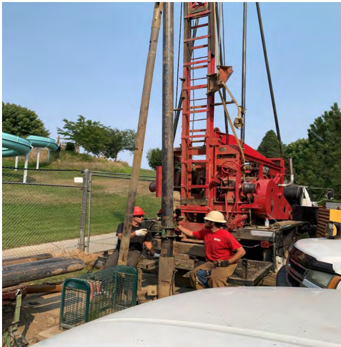
Repairs to Eagle Island Domestic Well
