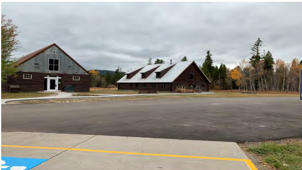
Road Paving and ADA Parking
