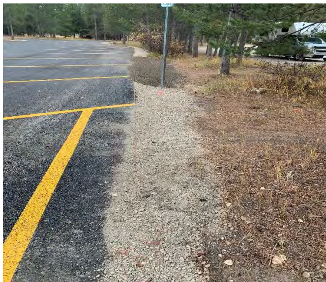
Finished parking lot and striping
