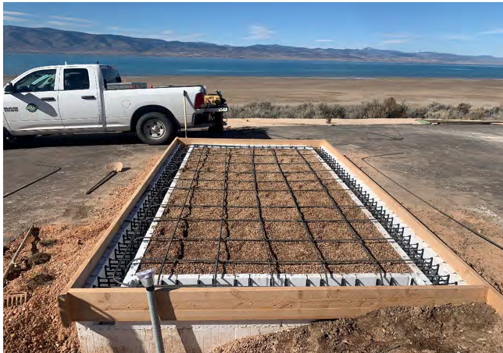
East Beach Kiosk Formwork
