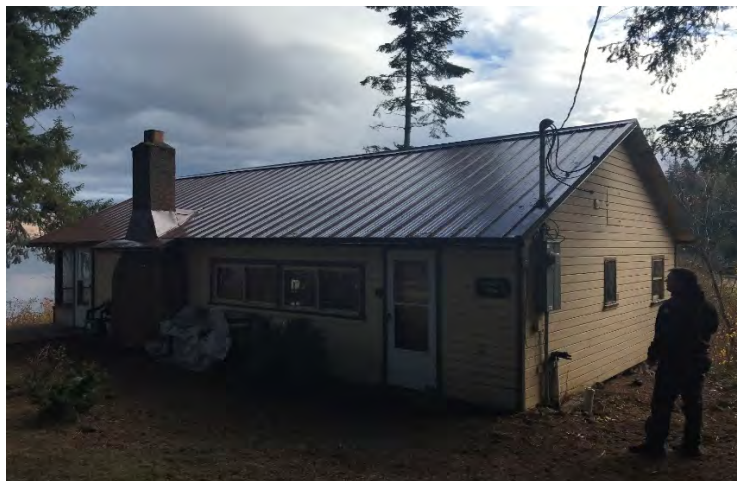
Heyburn Lakeview Cottage New Roof
