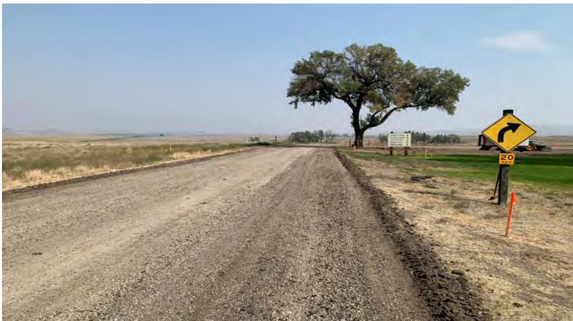
Bruneau Dunes access road milled and graded
