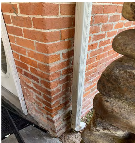
Castle Rocks VC Brick Repair
