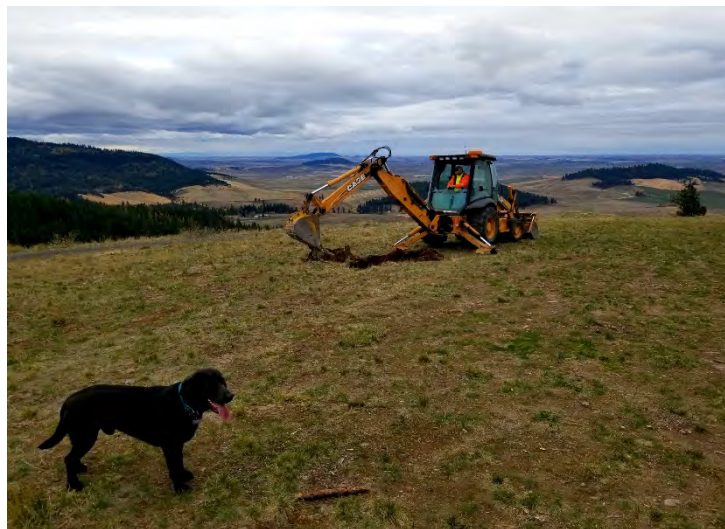
Digging test pits at potential future day use shelter
