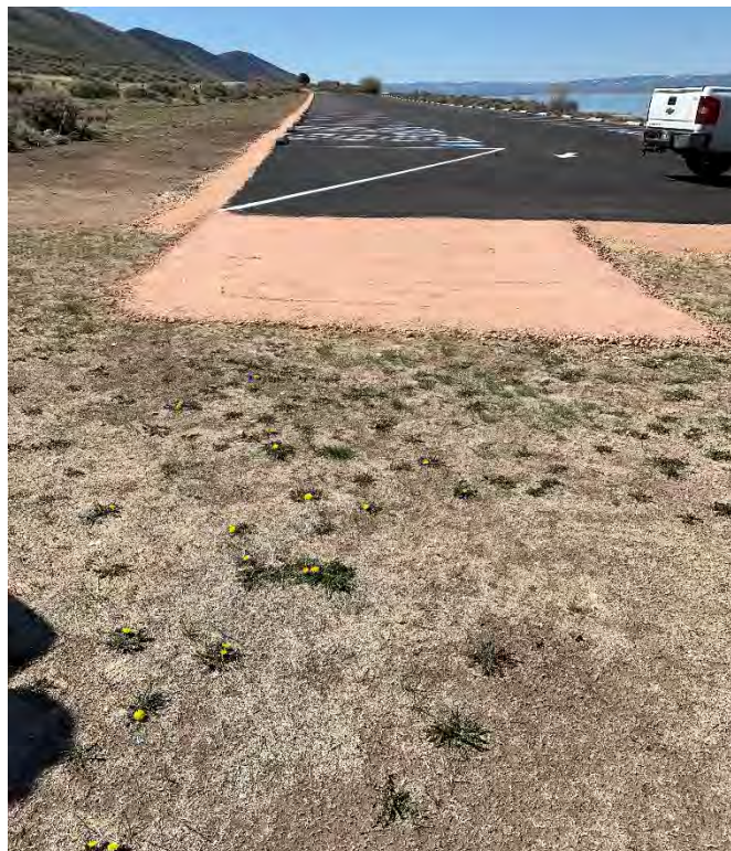
East Beach Paving Complete
