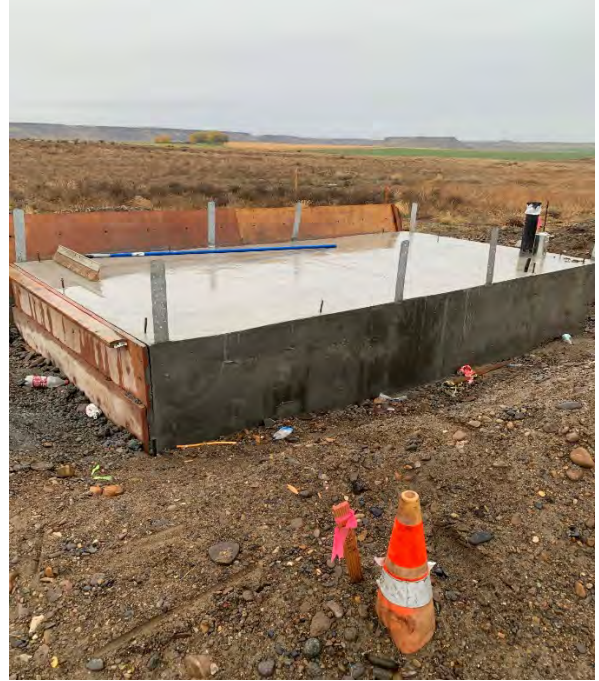
Slab on grade for new Kiosk
