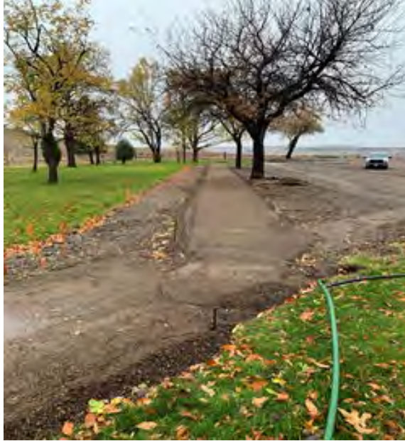
Sidewalk grading toward Kiosk
