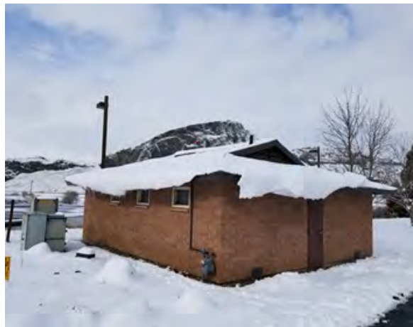
Hells Gate Remodel Marina Restroom
