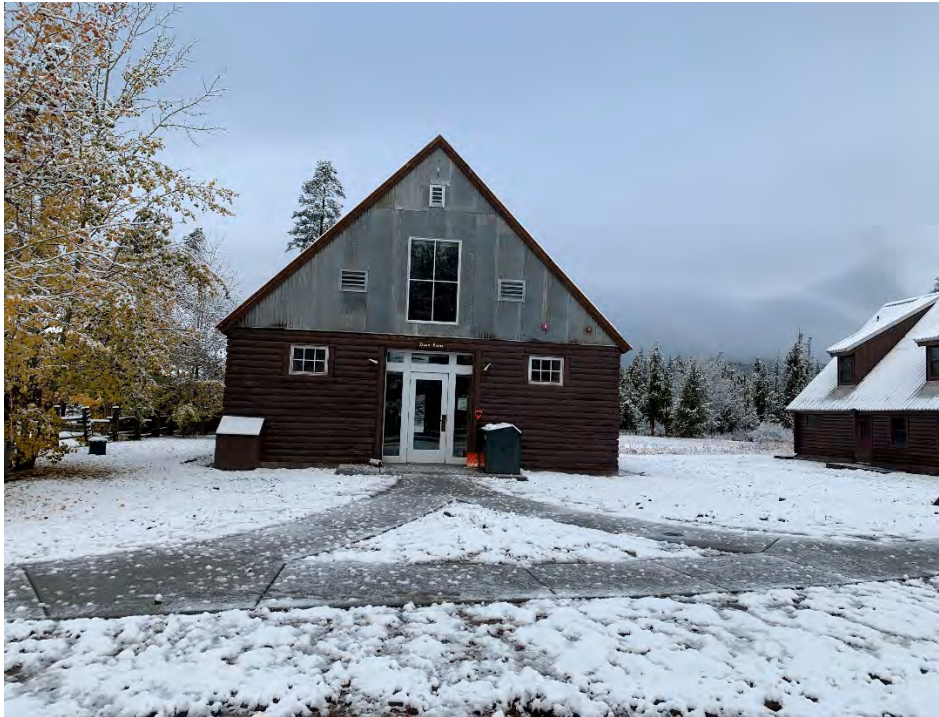
Poured sidewalks to buildings at Harriman
