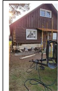
Log replacement work on the Cookhouse.
