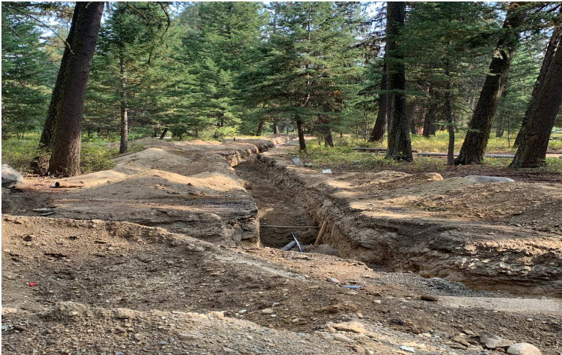
Ponderosa Aspen Loop trenches for water and electrical upgrades
