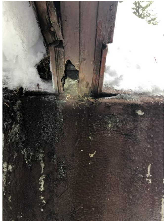
FIGURE 4: Water damage at truss-to-concrete-pier connection
