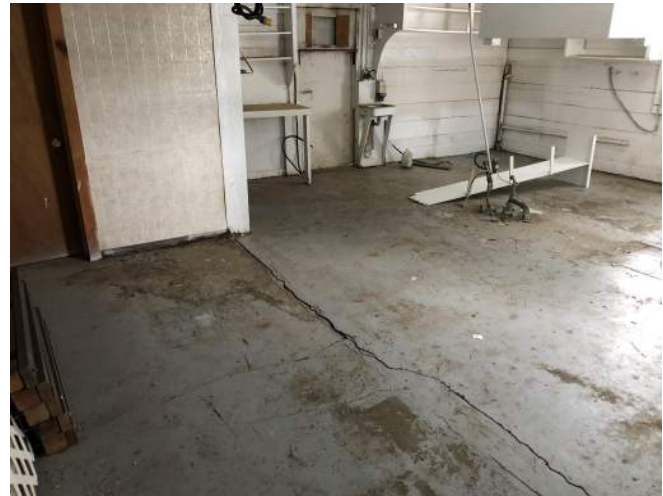
FIGURE 12: Crack at connection between western and main portion of the building
