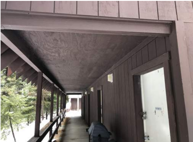
FIGURE 7: Posts and beams at front porch
