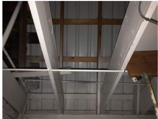
FIGURE 14: Roof framing at the addition
