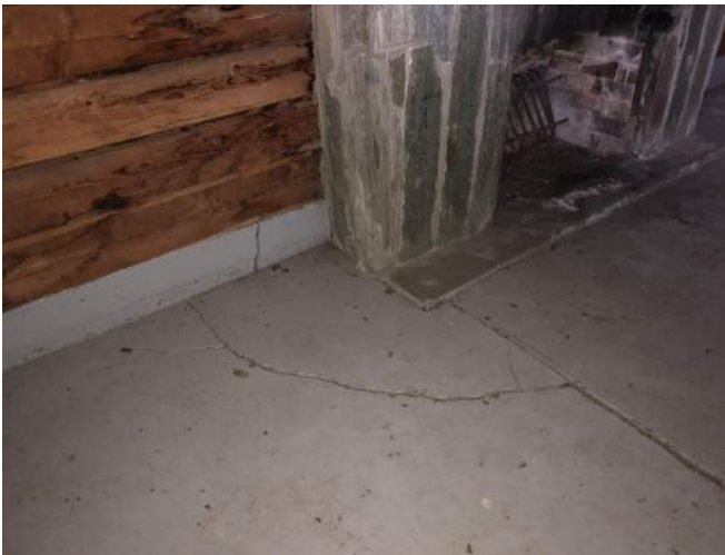
FIGURE 13: Crack in main portion at the slab and foundation wall
