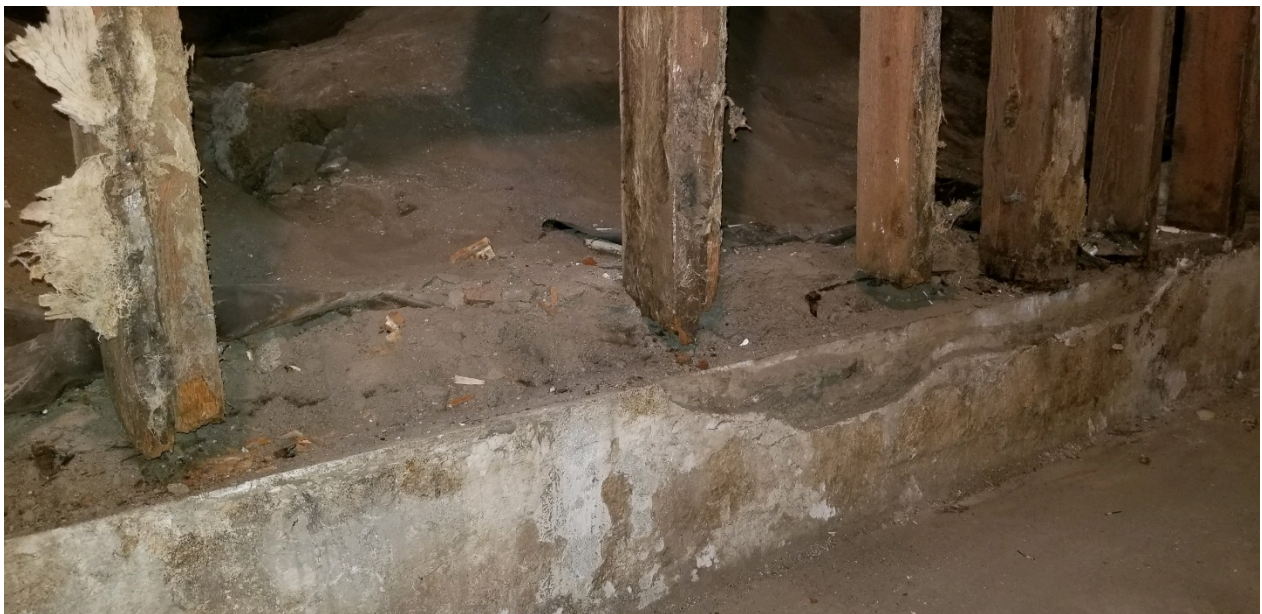
Jones House Mold Remediation, non-existent sill plate on foundation
