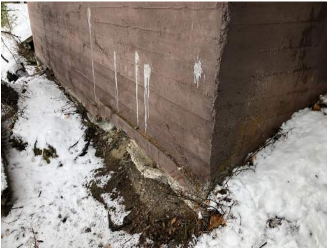
FIGURE 11: Soil erosion at western portion
