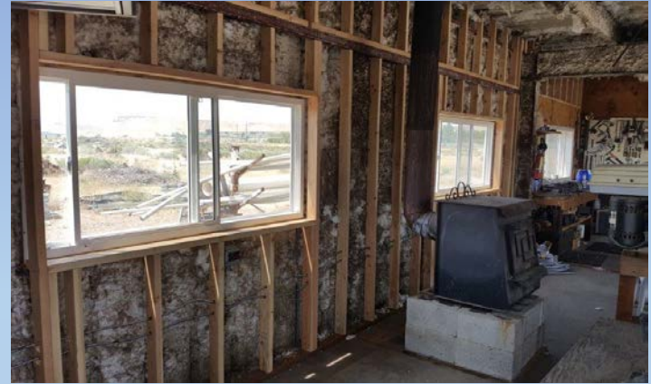
DPW Project: Upgrades to the shop including new windows, garage doors, insulated new roof
