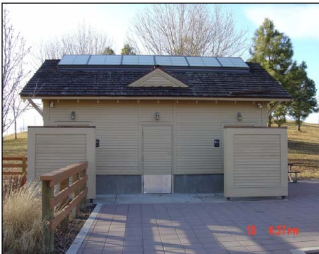
1.a East side restroom
