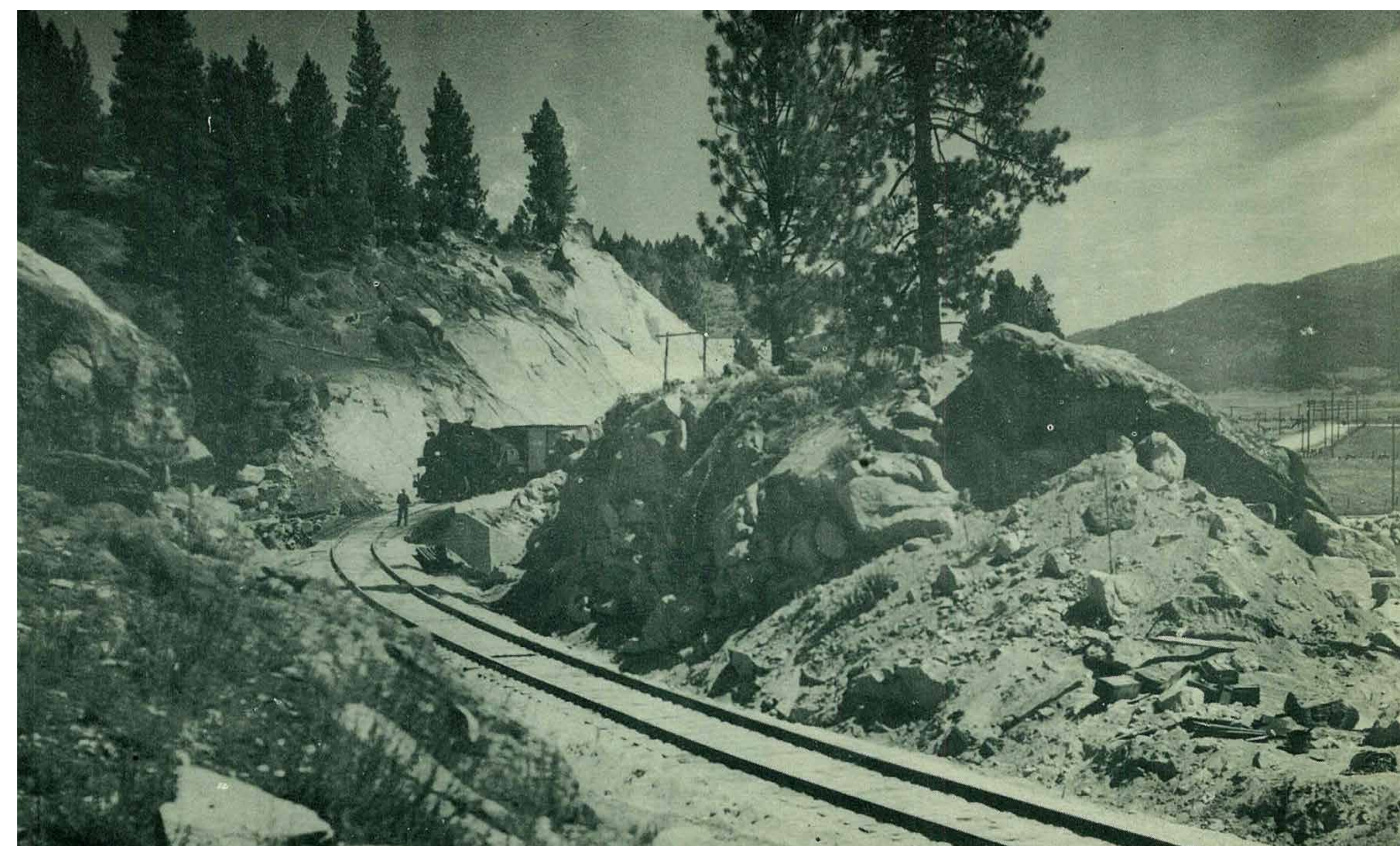
Cascade Dam Railroad Relocation. First train over new track. July 1947.
