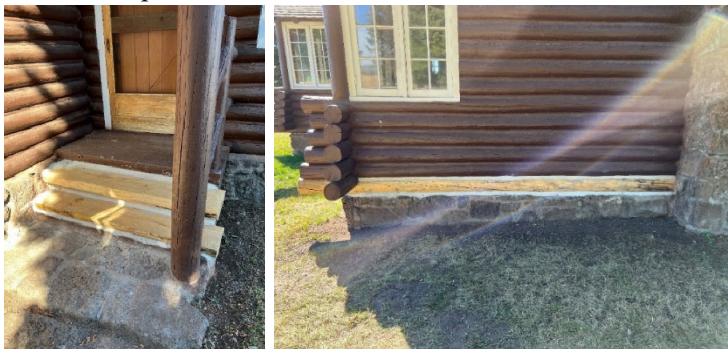
Log replacement and window work on the Ranch Office
