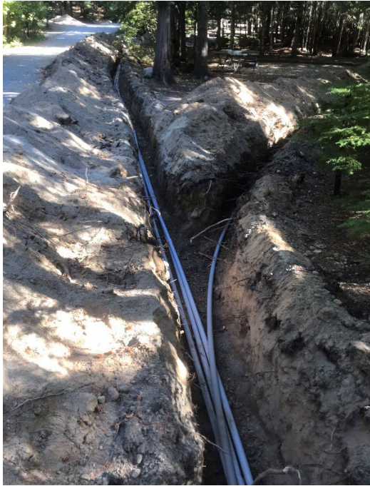
Priest Lake Campground Electrical Upgrades
