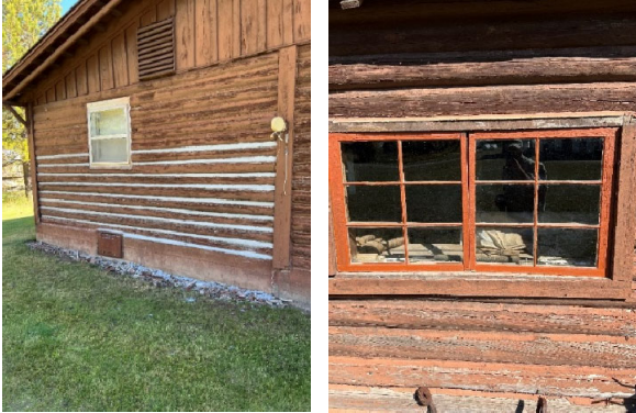
Small shop window replacements
