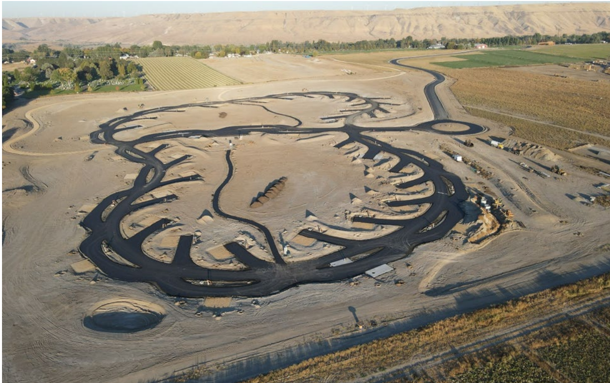
Billingsley Creek Campground and Entrance Road Paved
