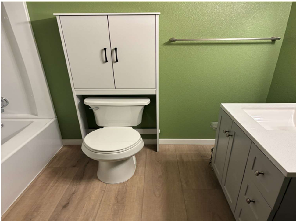
Thousand Springs Manager's House Bathroom Upgrades
