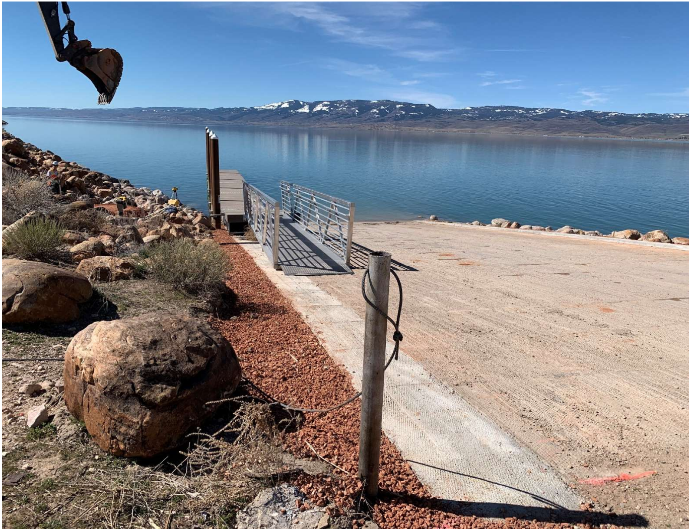
Bear Lake N. Beach Boat Ramp Replacement
