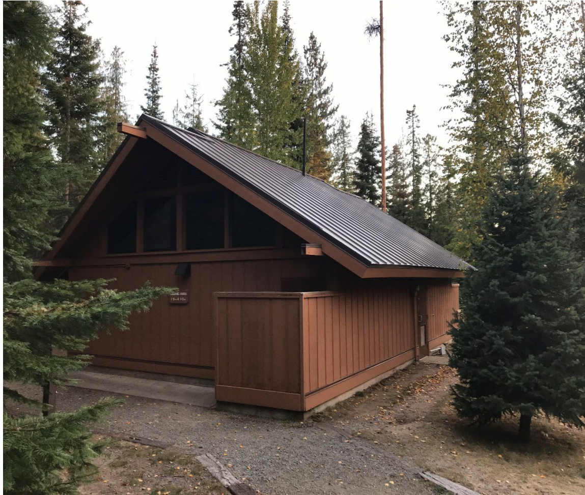
Priest Lake New Roof on Shower House
