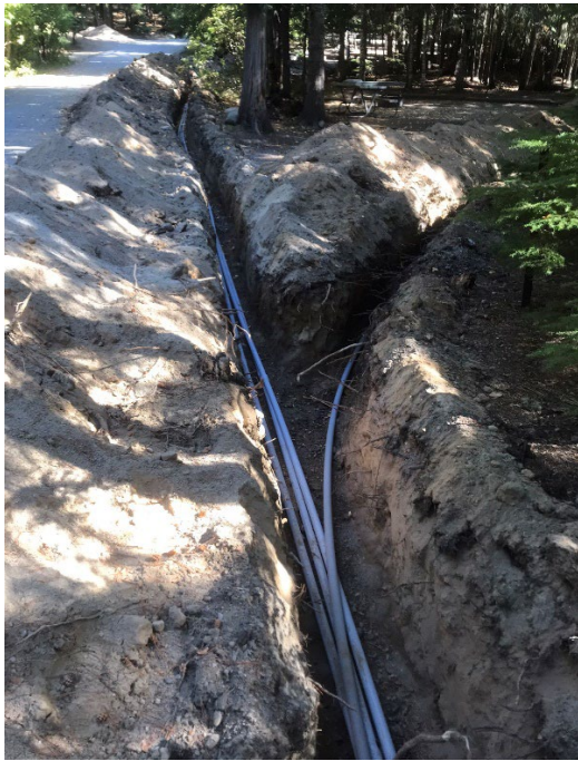
Priest Lake Campground Electrical Upgrades
