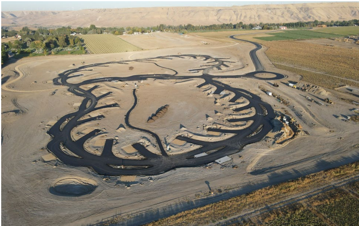
Billingsley Creek Campground and Entrance Road Paved
