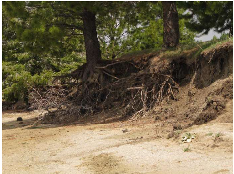
Eroded shoreline at Lake Cascade will be restored with a FY 2025 project.
