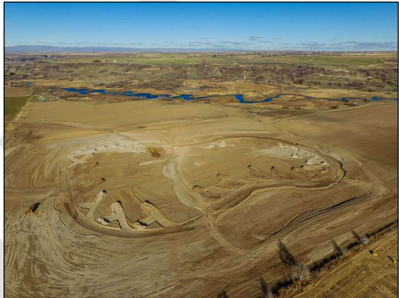
Billingsley Creek Campground under construction at Thousand Springs State Park, partially funded by a LWCF grant.
