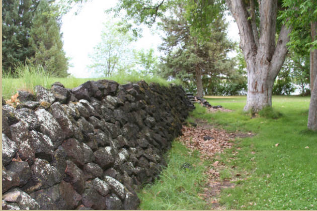
One of the rock walls built by the CCC at Lake Walcott State Park
