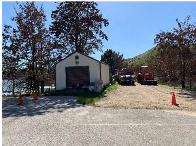
Marina Equipment Storage and Barn
