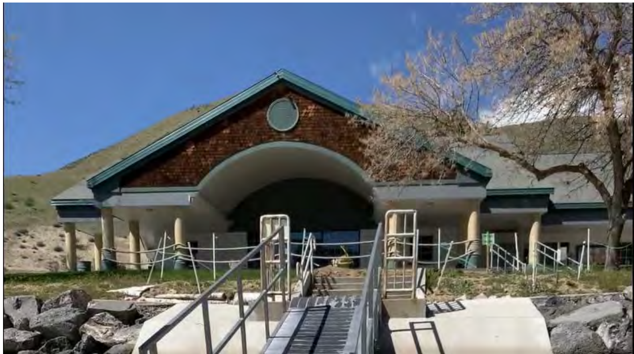
Spring Shores Marina Boater Services Building
