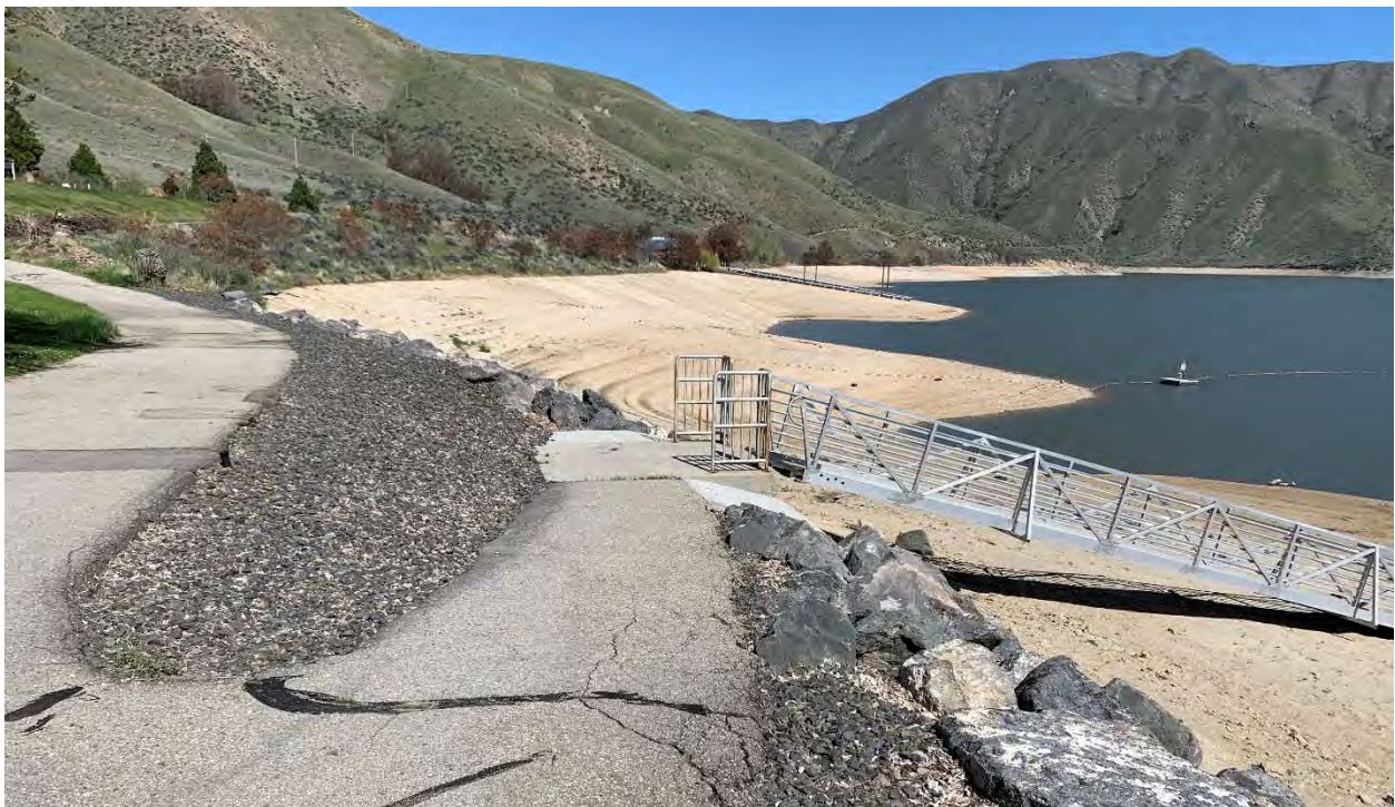
Typical Accessible Concrete Abutment
