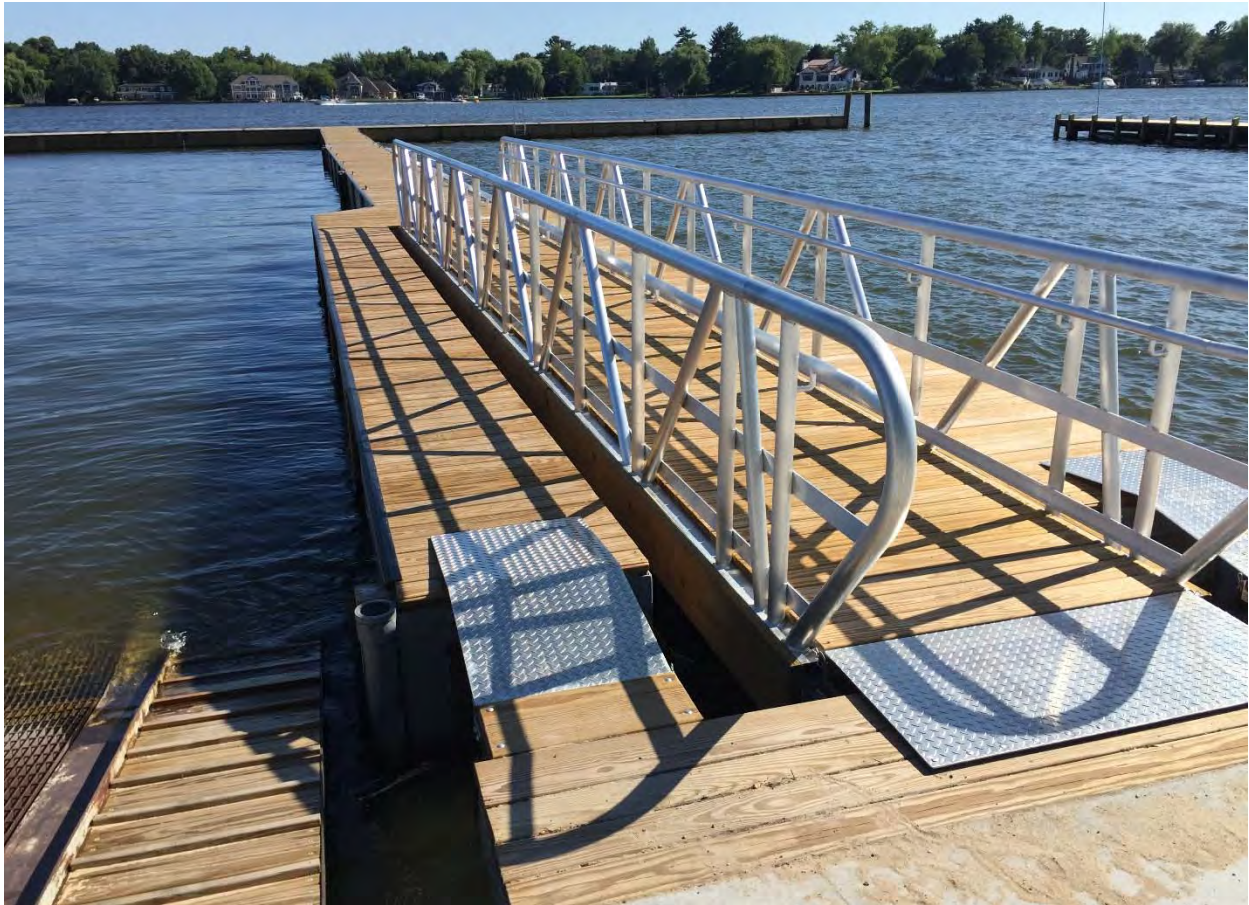
Typical Floating Wave Attenuator
