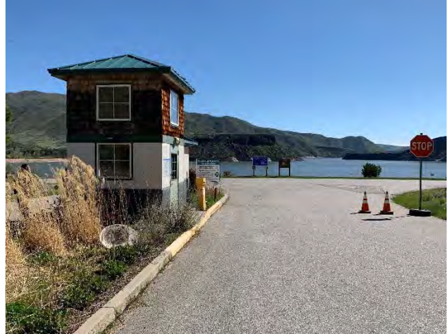
Marina Entry Gate House
