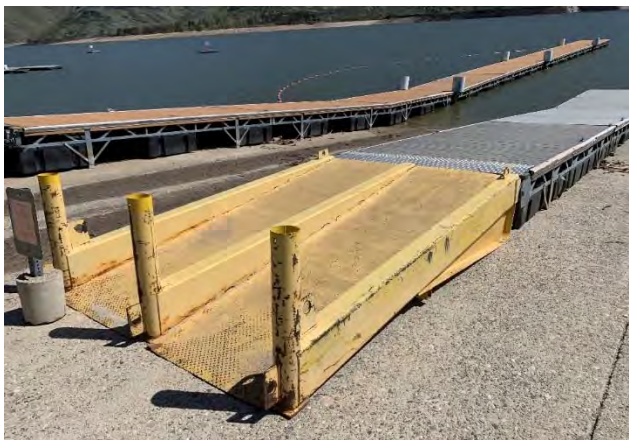
ADA Compliant Skid Pier Access
