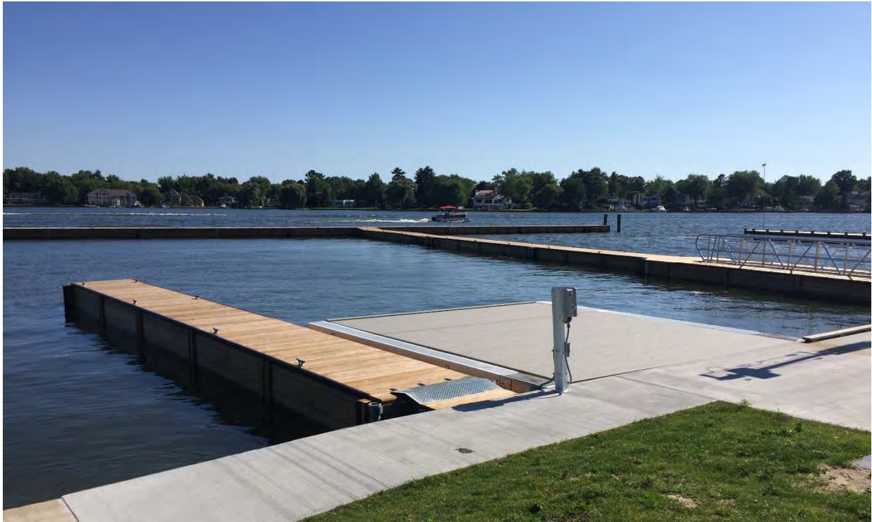
Typical Floating Wave Attenuator
