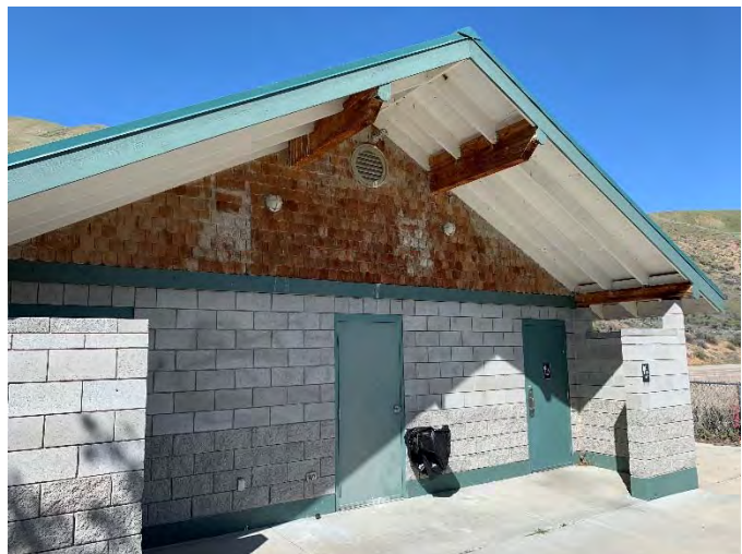
East Boat Launch Restrooms
