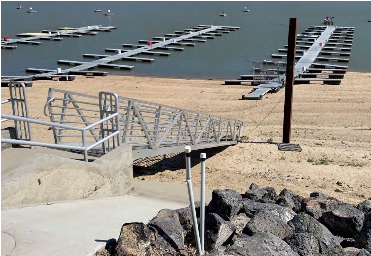
Typical Abutment and Anchorage System
