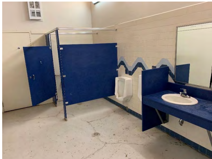
Interior View of Boater Restrooms
