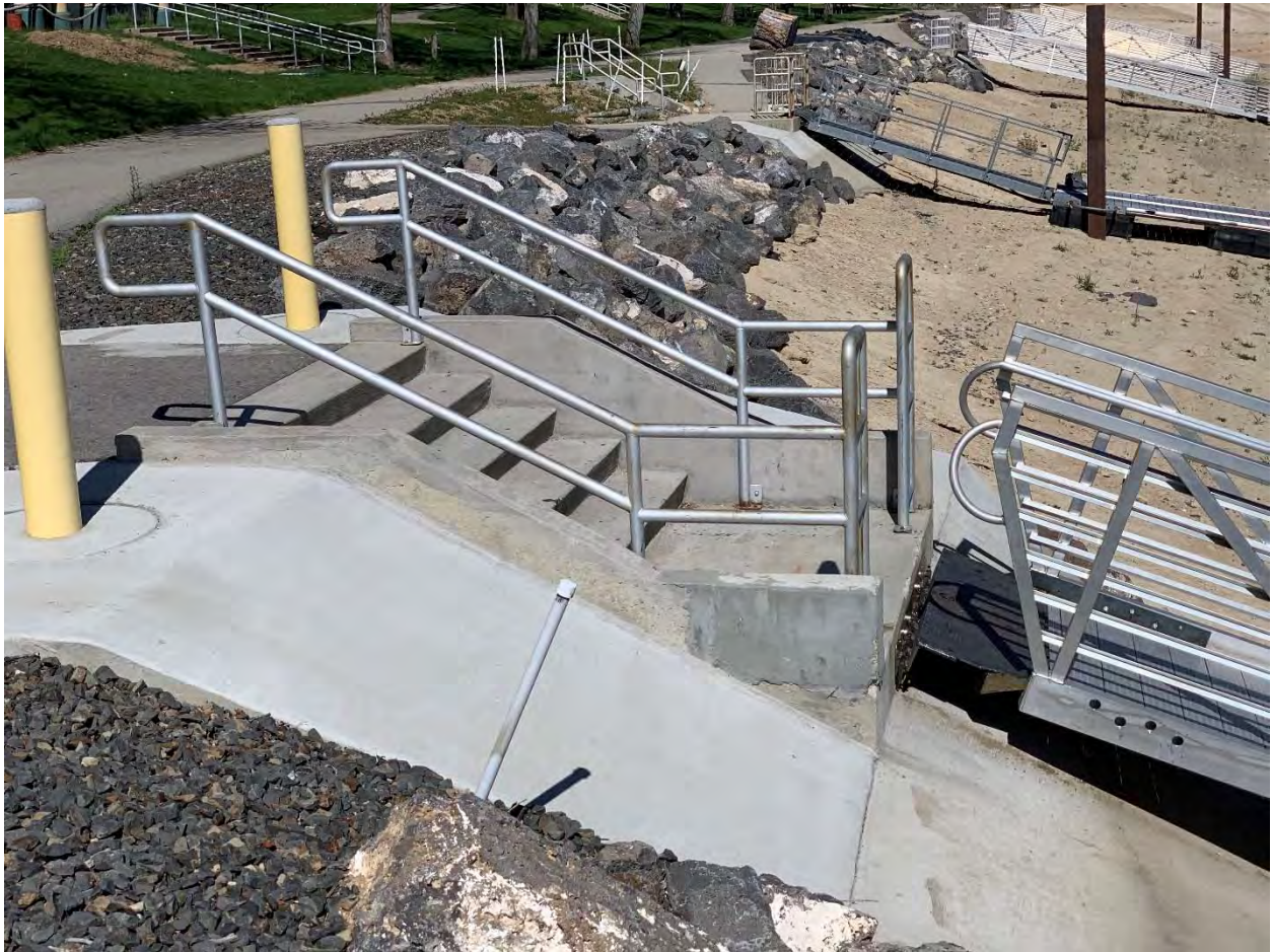
Typical Non-Accessible Concrete Abutment With Steps
