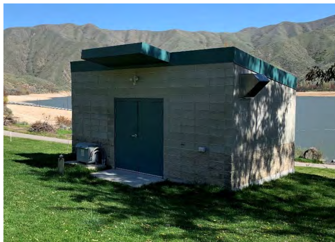
Potable Water Pumping Facility
