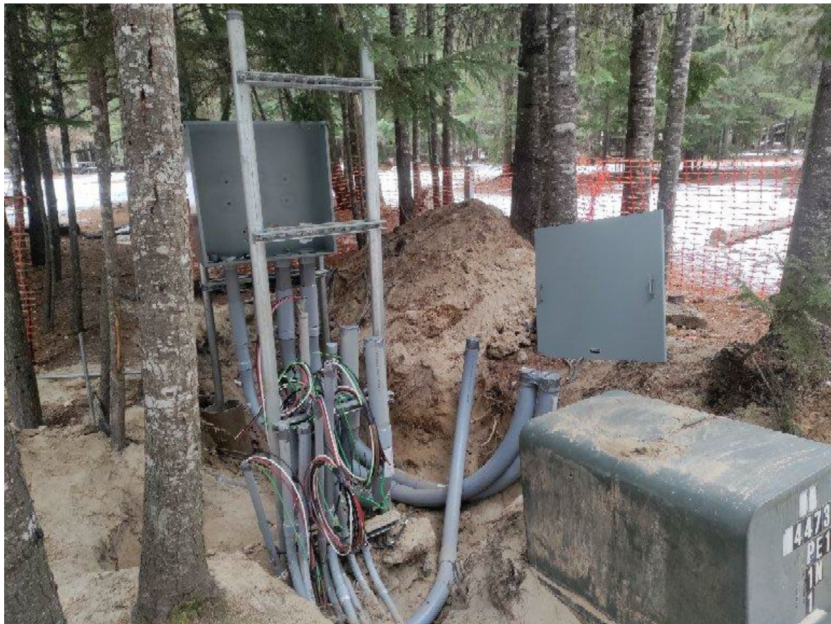
Priest Lake Campground Electrical Upgrades
