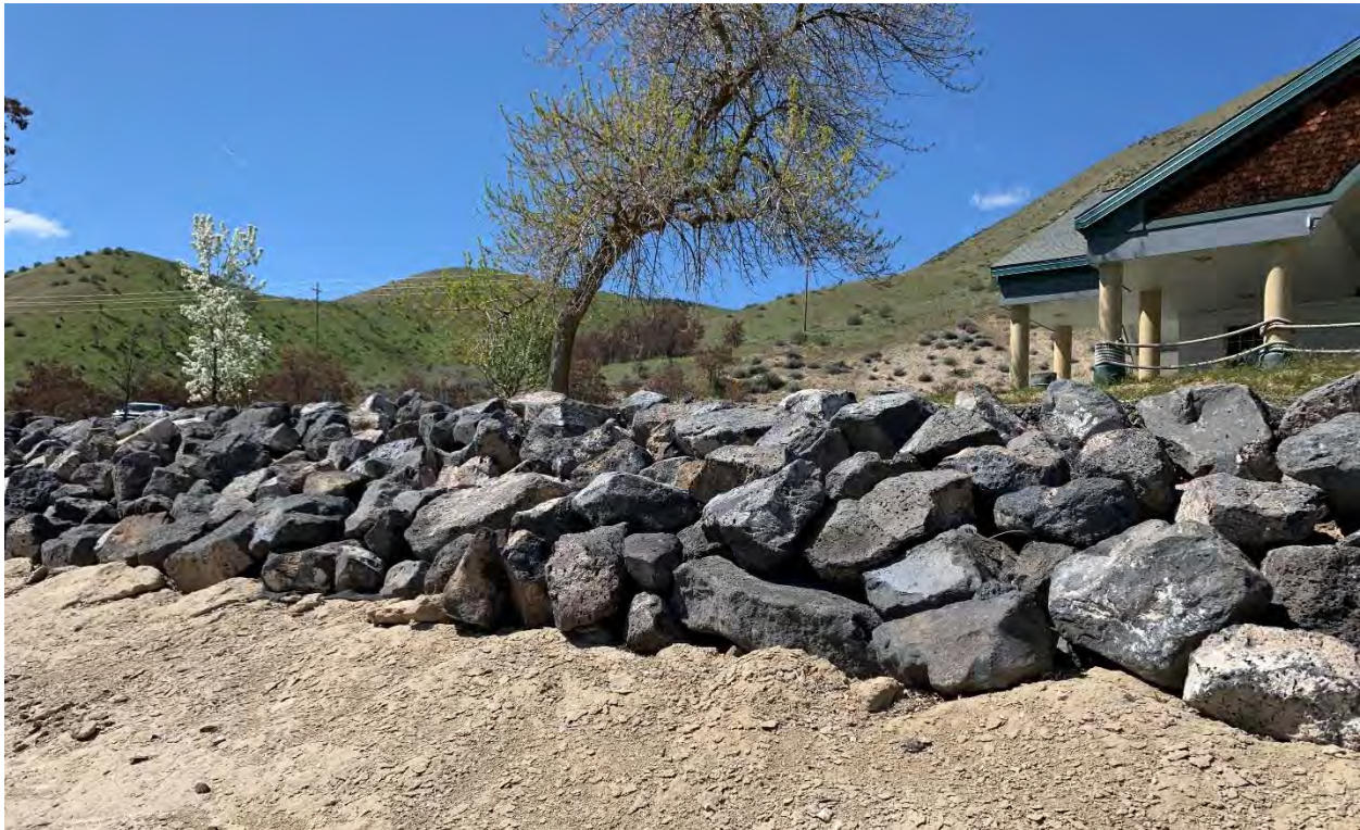
Typical Rock Revetment along the Northern Portion of Marina
